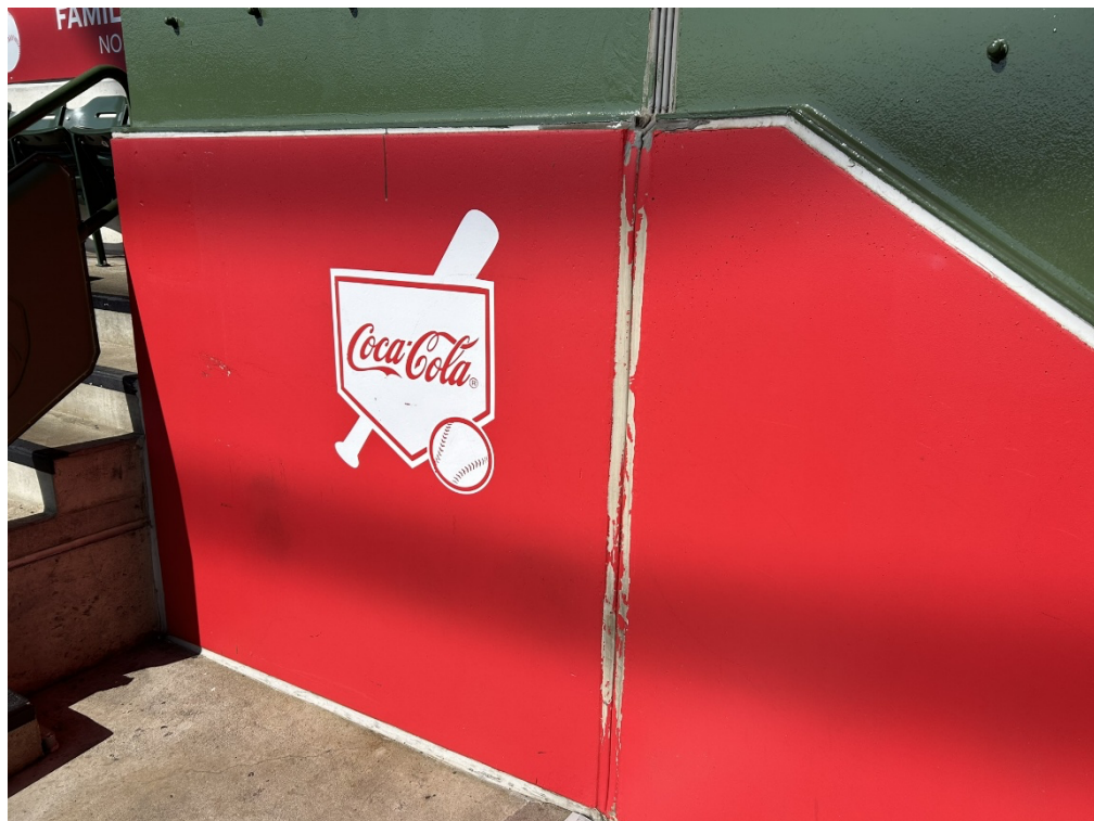
Photo 6-Section 417 Expansion Joint
