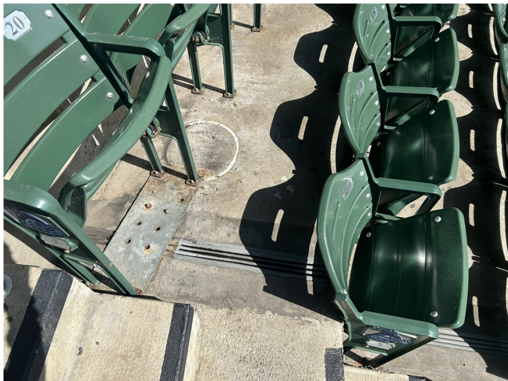
Photo 2-Section 417 Expansion Joint
