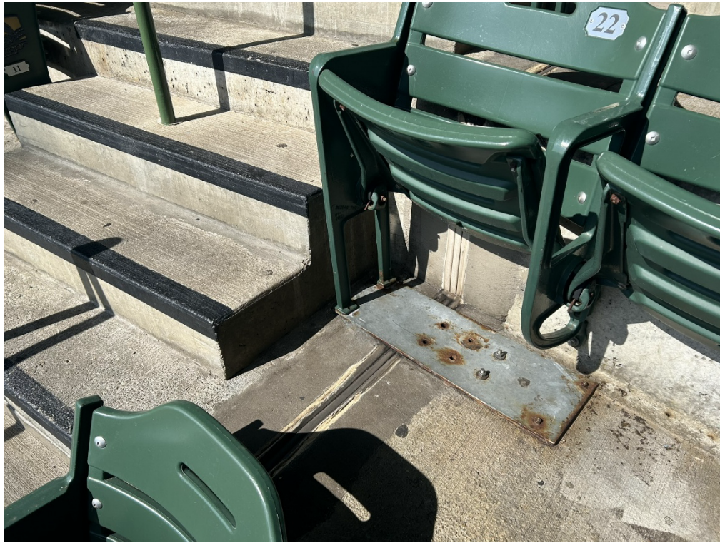
Photo 3-Section 417 Expansion Joint
