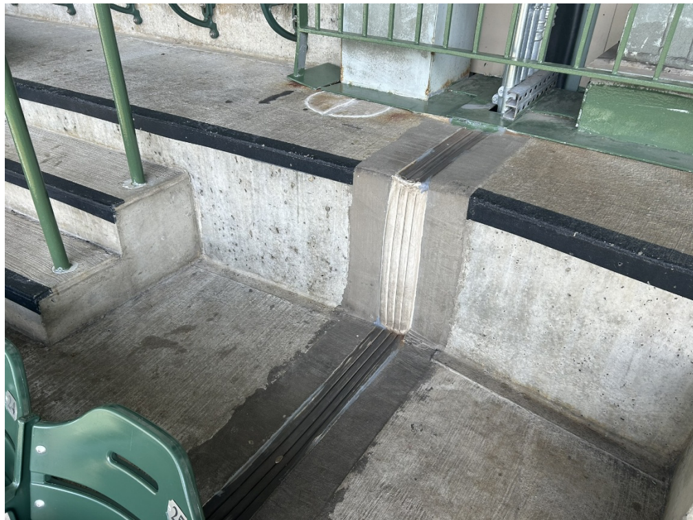
Photo 14-Section 426 Expansion Joint
