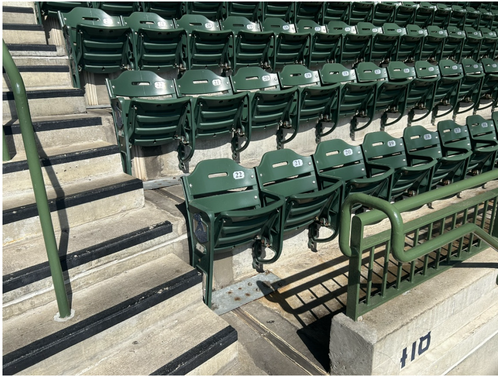
Photo 1-Section 417 Expansion Joint
