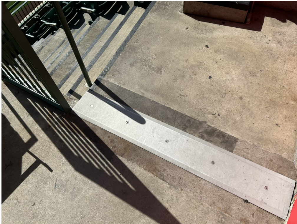
Photo 7-Section 417 Expansion Joint
