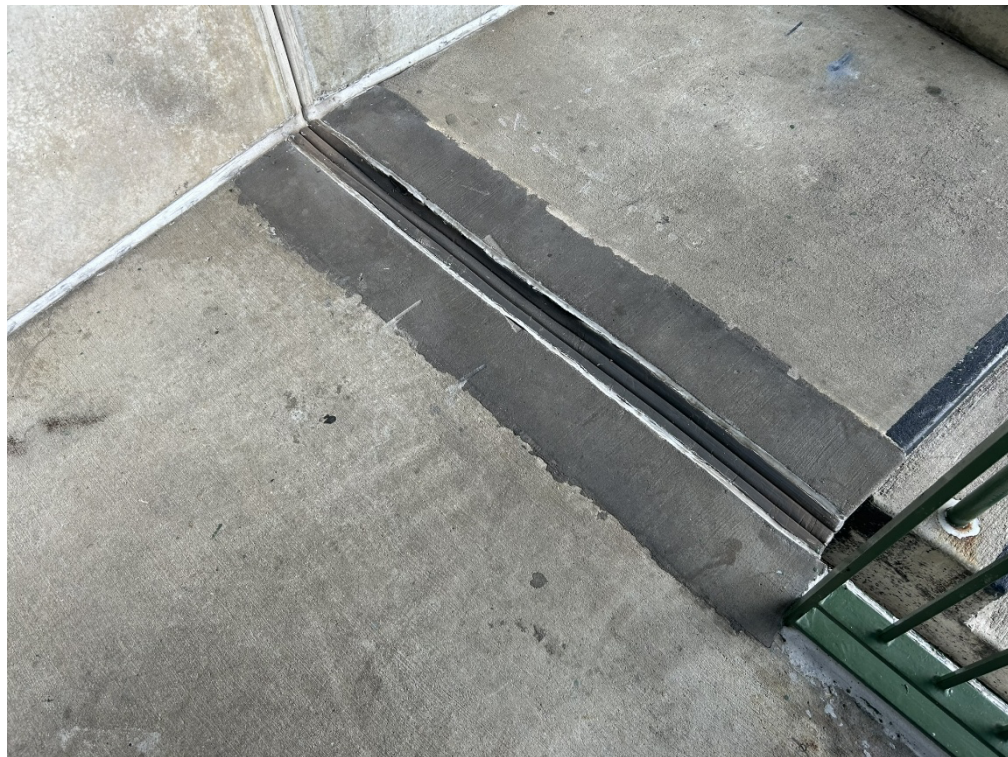
Photo 12-Section 426 Expansion Joint
