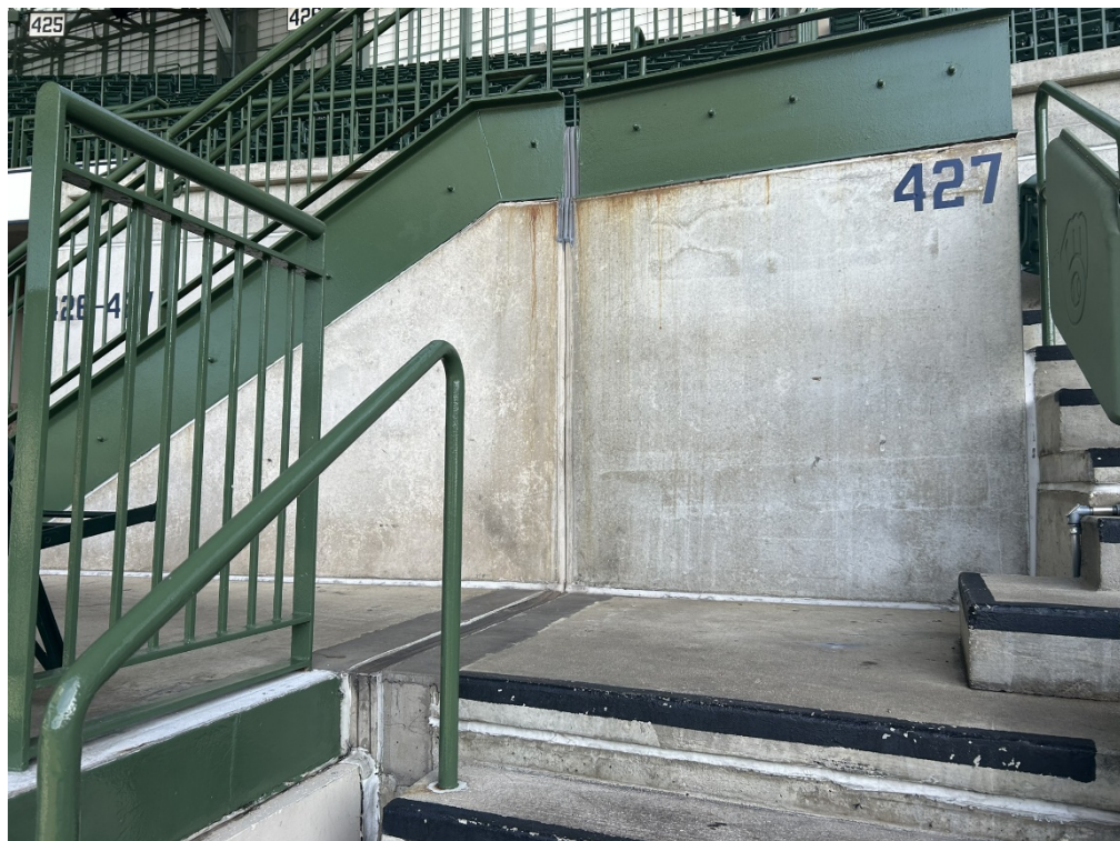
Photo 10-Section 426 Expansion Joint
