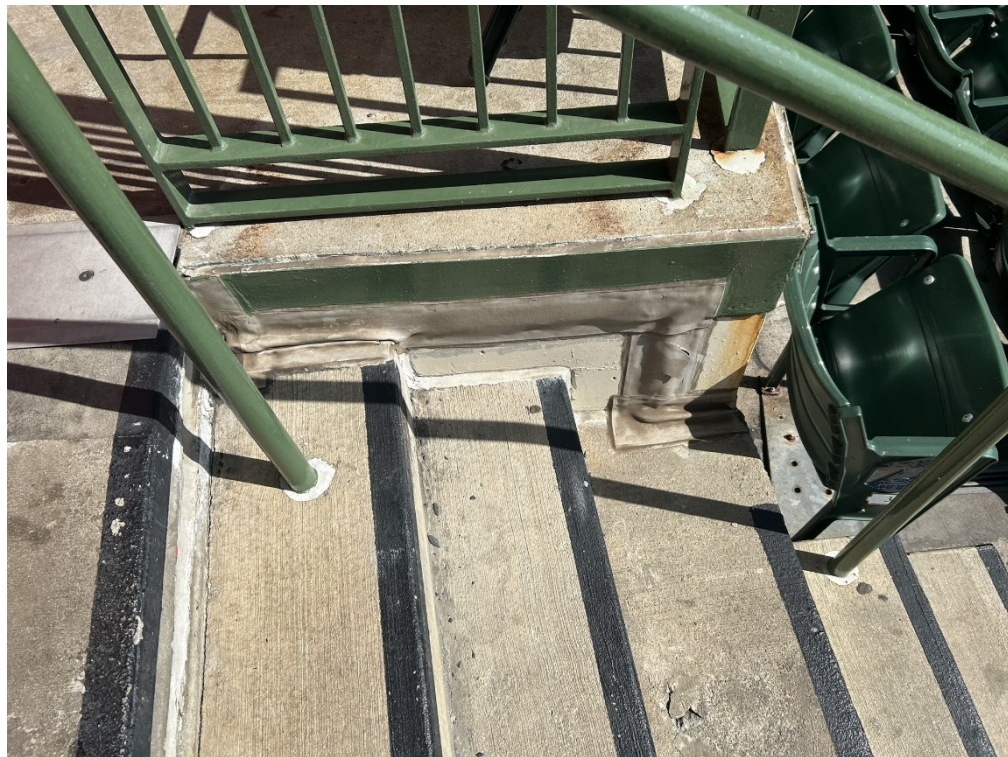
Photo 4-Section 417 Expansion Joint
