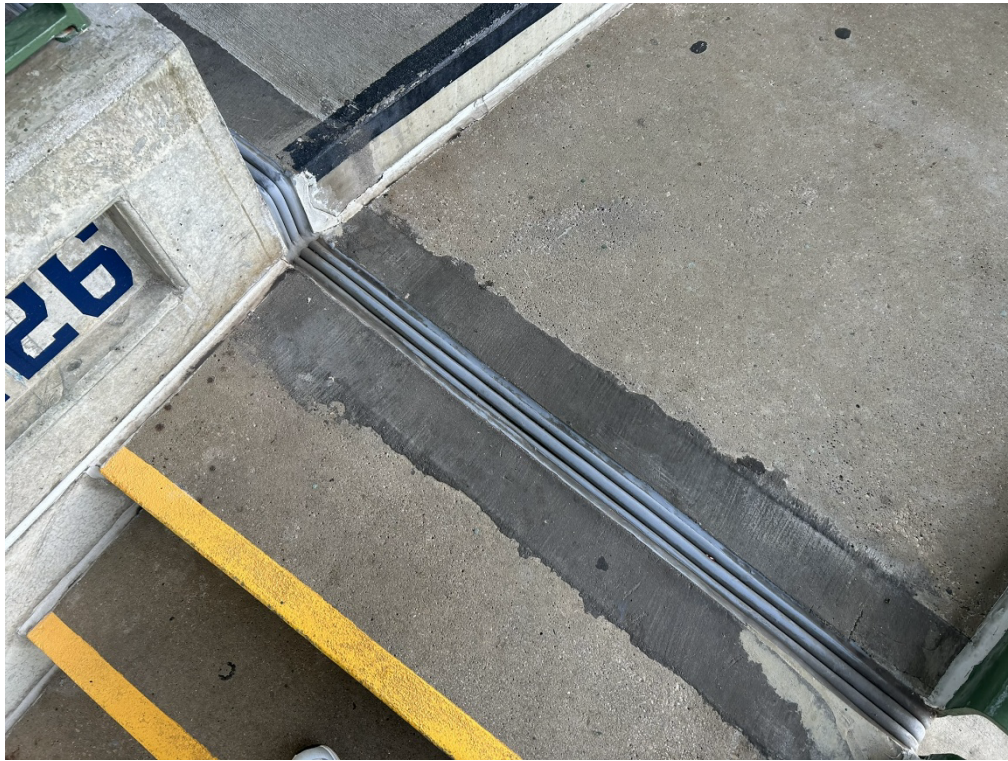
Photo 11-Section 426 Expansion Joint
