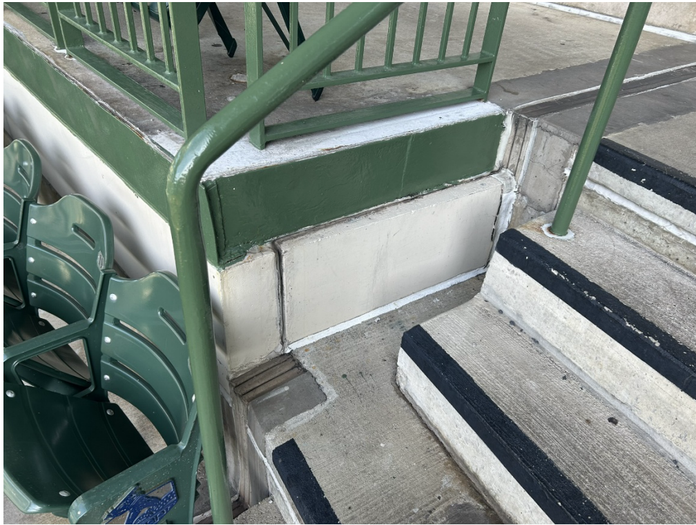
Photo 13-Section 426 Expansion Joint
