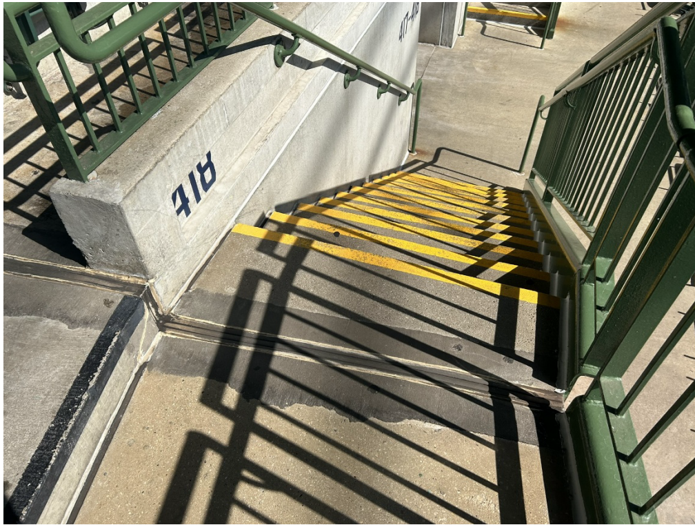
Photo 5-Section 417 Expansion Joint
