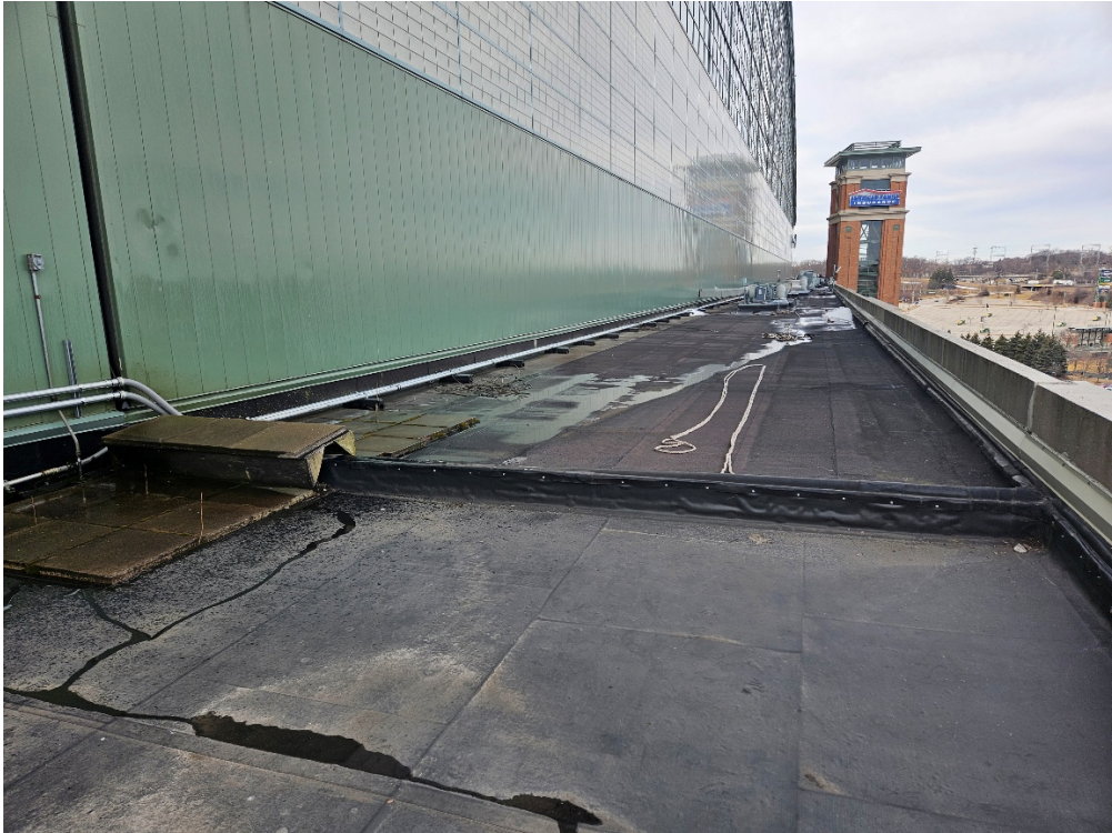
Photo 1- Flat Roof Expansion Joint
