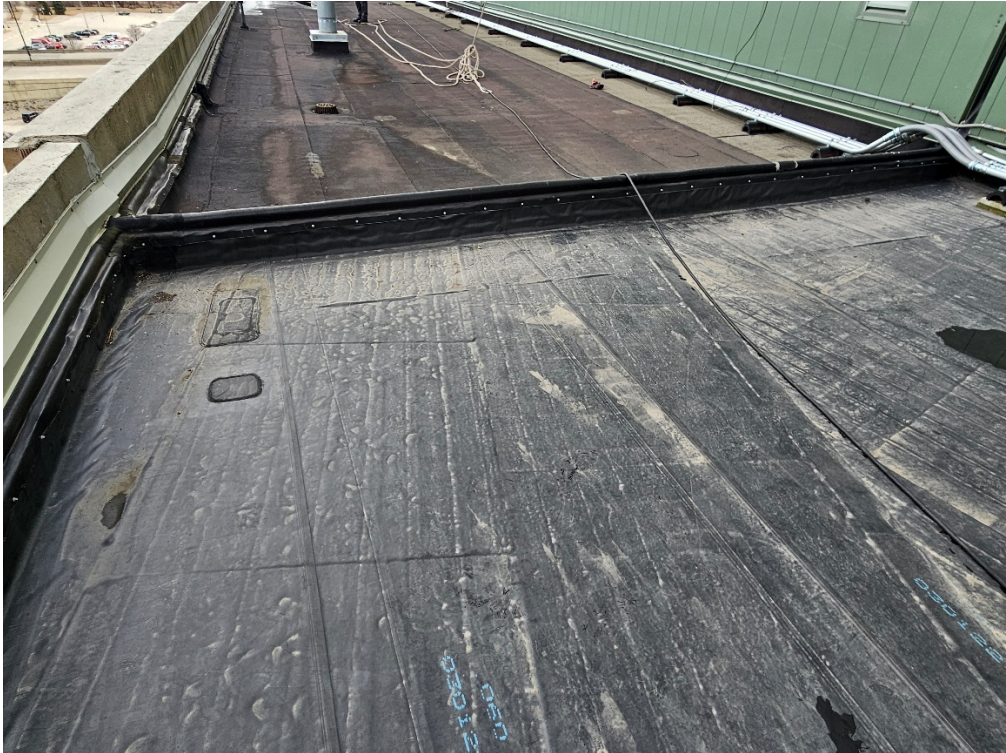
Photo 2- Flat Roof Expansion Joint
