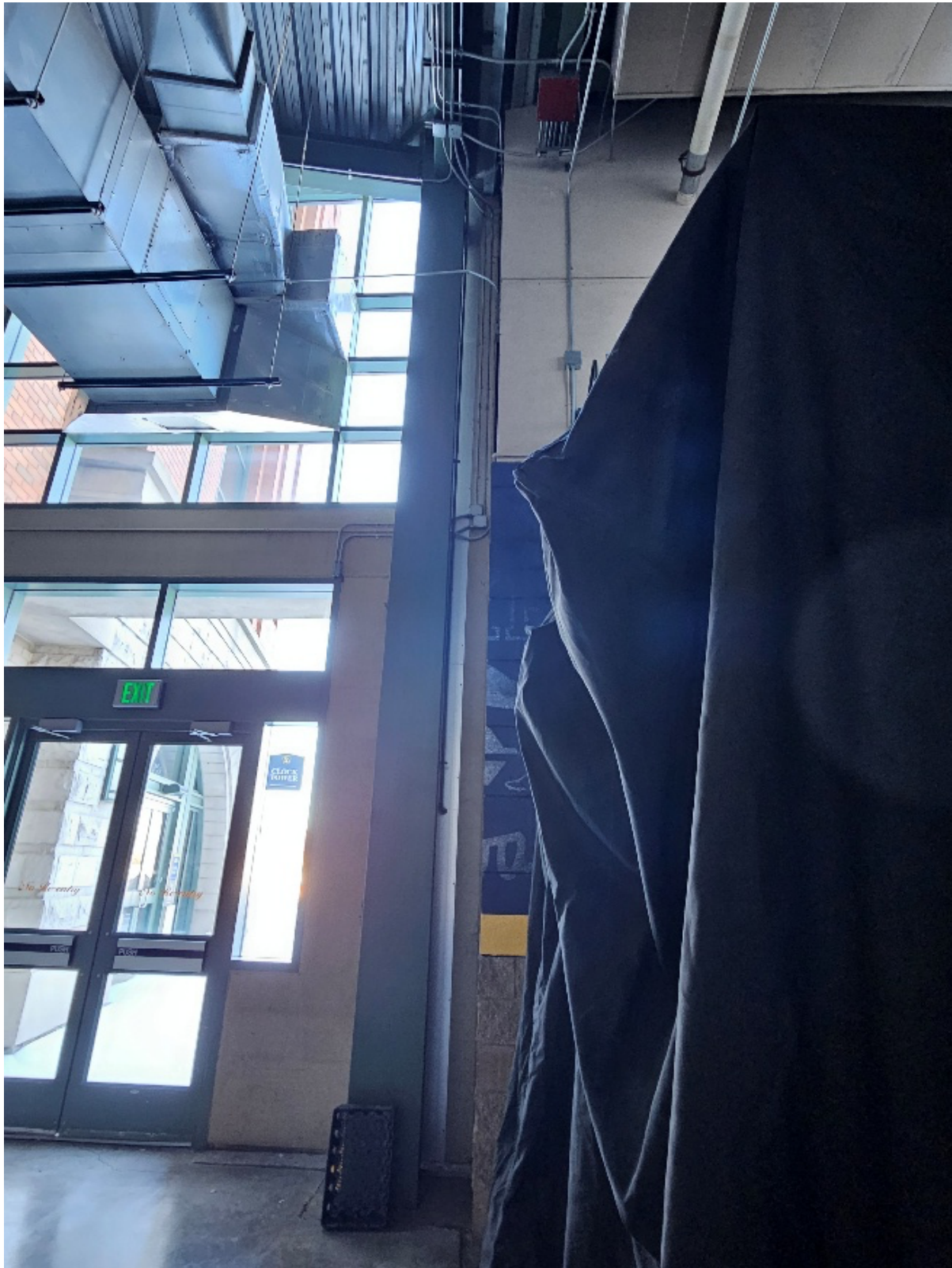
Photo 4-Left Field Tower Field Level
