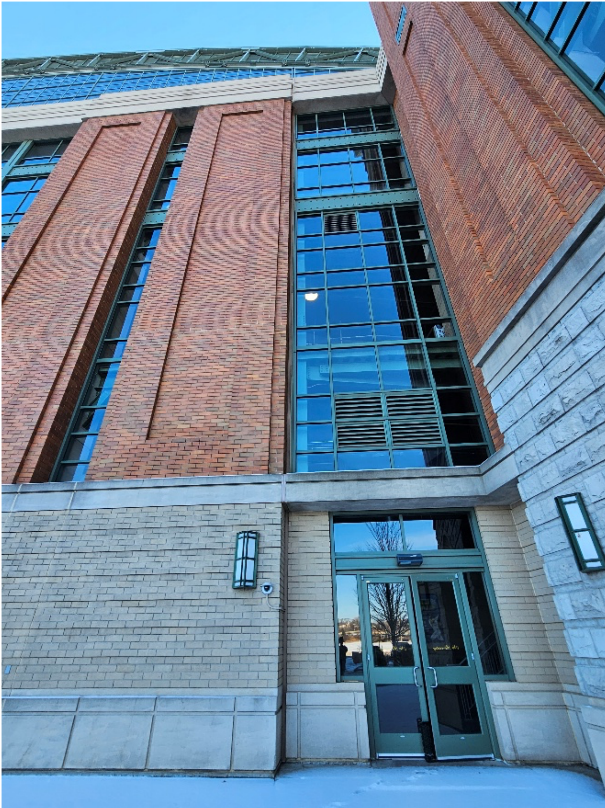
Photo 6-Left Field Tower Exterior
