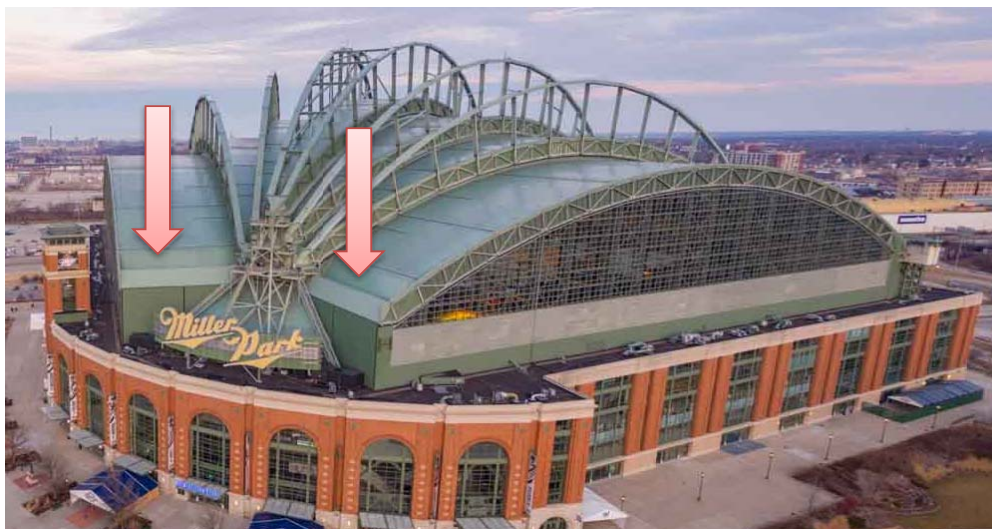
Figure II – Elevation Photo of Gutter
