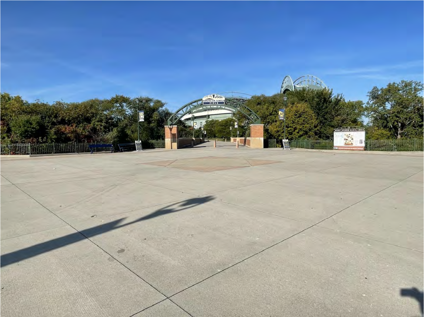
Photo 18: Uecker/Yount Lot: Concrete paved plaza and pedestrian path along west side of Uecker and Yount Lots: 6-inch concrete pavement overlying 8-inches crushed aggregate. Photo taken facing west on October 4, 2022.
