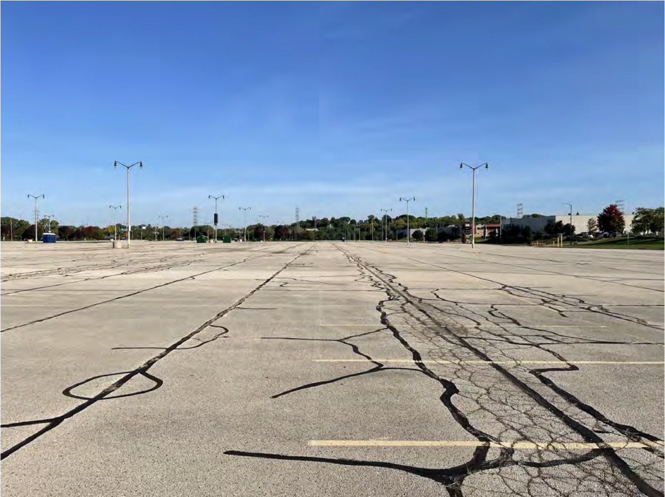
Photo 10: Uecker Lot: Asphalt cap over Uecker Lot: 4-inch asphalt pavement overlying 8-inches of crushed aggregate base course. Photo taken facing north on October 4, 2022.
