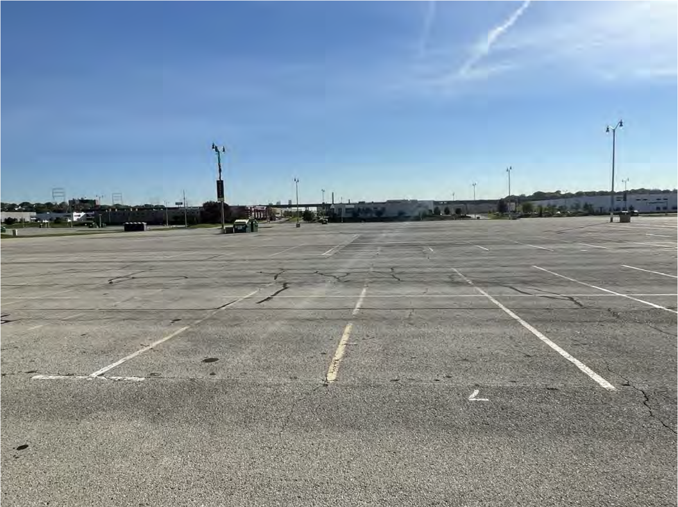
Photo 17: Uecker Lot: Asphalt cap over Uecker Lot: 4-inch asphalt pavement overlying 8-inches of crushed aggregate base course. Photo taken facing east on October 4, 2022.
