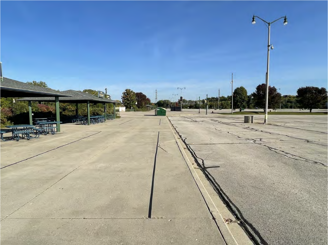
Photo 16: Uecker Lot: Concrete paved plaza and pedestrian path along west side of Uecker Lot (shown on left side of photo): 6-inch concrete pavement overlying 8-inches crushed aggregate. Asphalt paved Uecker Lot (shown on right side of photo): 4-inch asphalt pavement overlying 8-inches crushed aggregate. Photo taken facing north on October 4, 2022.
