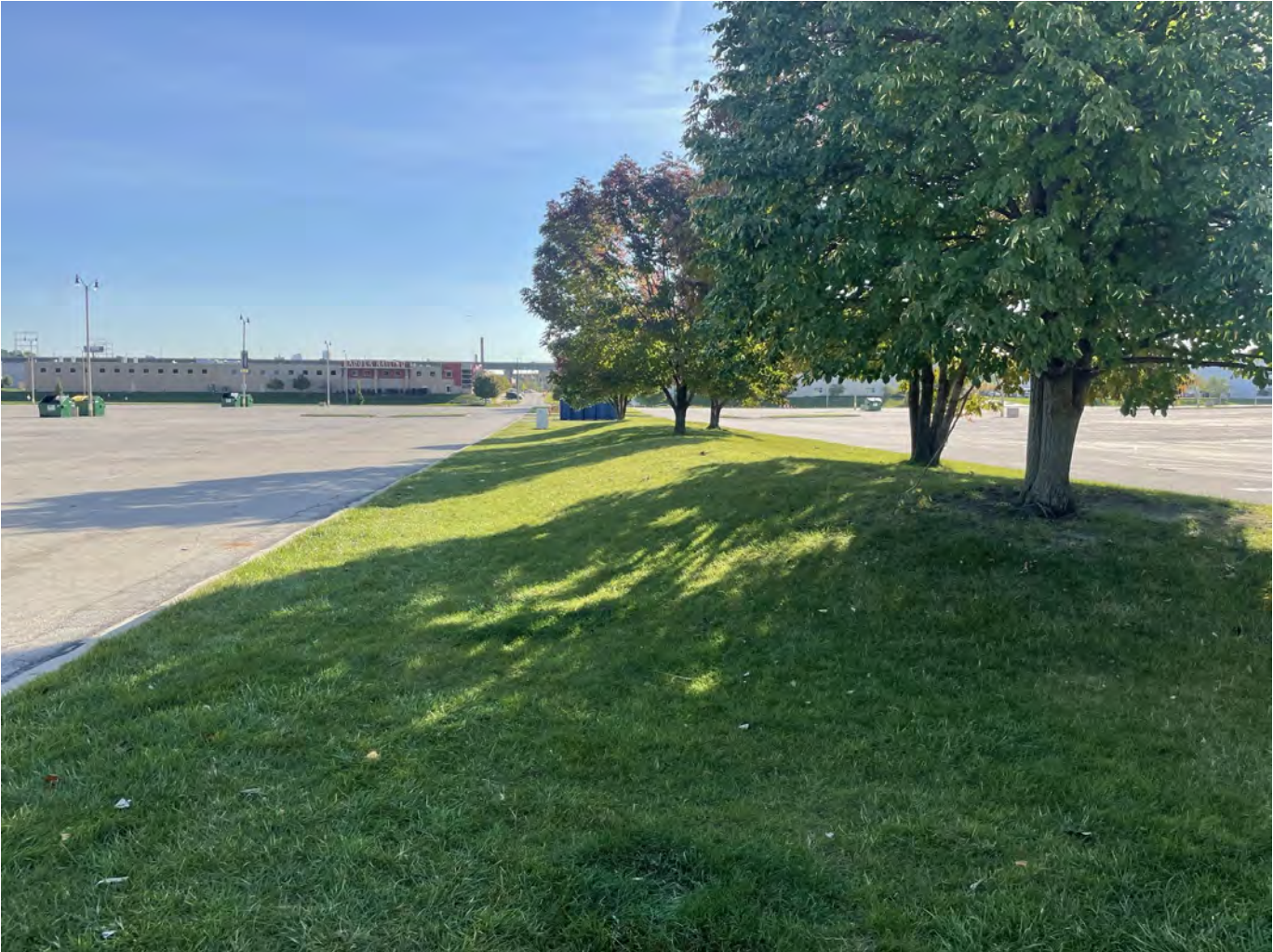
Photo 19: Uecker/Yount Lot: Greenspace cap parking lot island/median between Yount and Uecker Lots on west side of site: 12-inches of low permeability non-impacted soil covered with 4-inches of vegetated topsoil (grass) as well as various landscape plantings.
