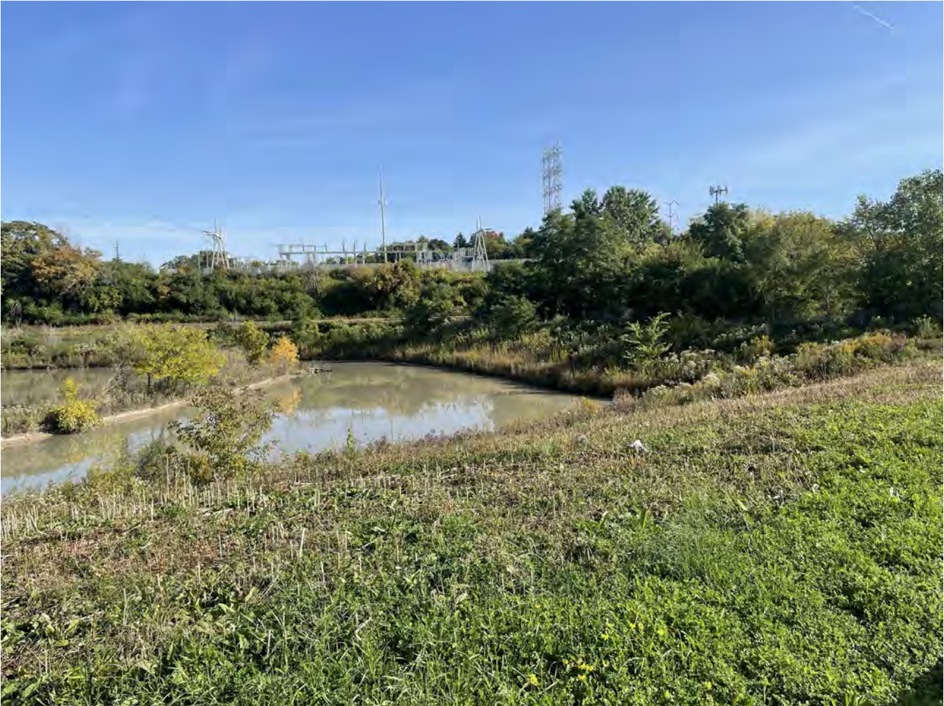
Photo 24: Yount Lot: Storm water pond with clay liner and geomembrane liner, north of Yount Lot and Selig Drive. Landscaping around the pond consists of vegetated topsoil with native plantings. Photo taken facing north on October 4, 2022.
