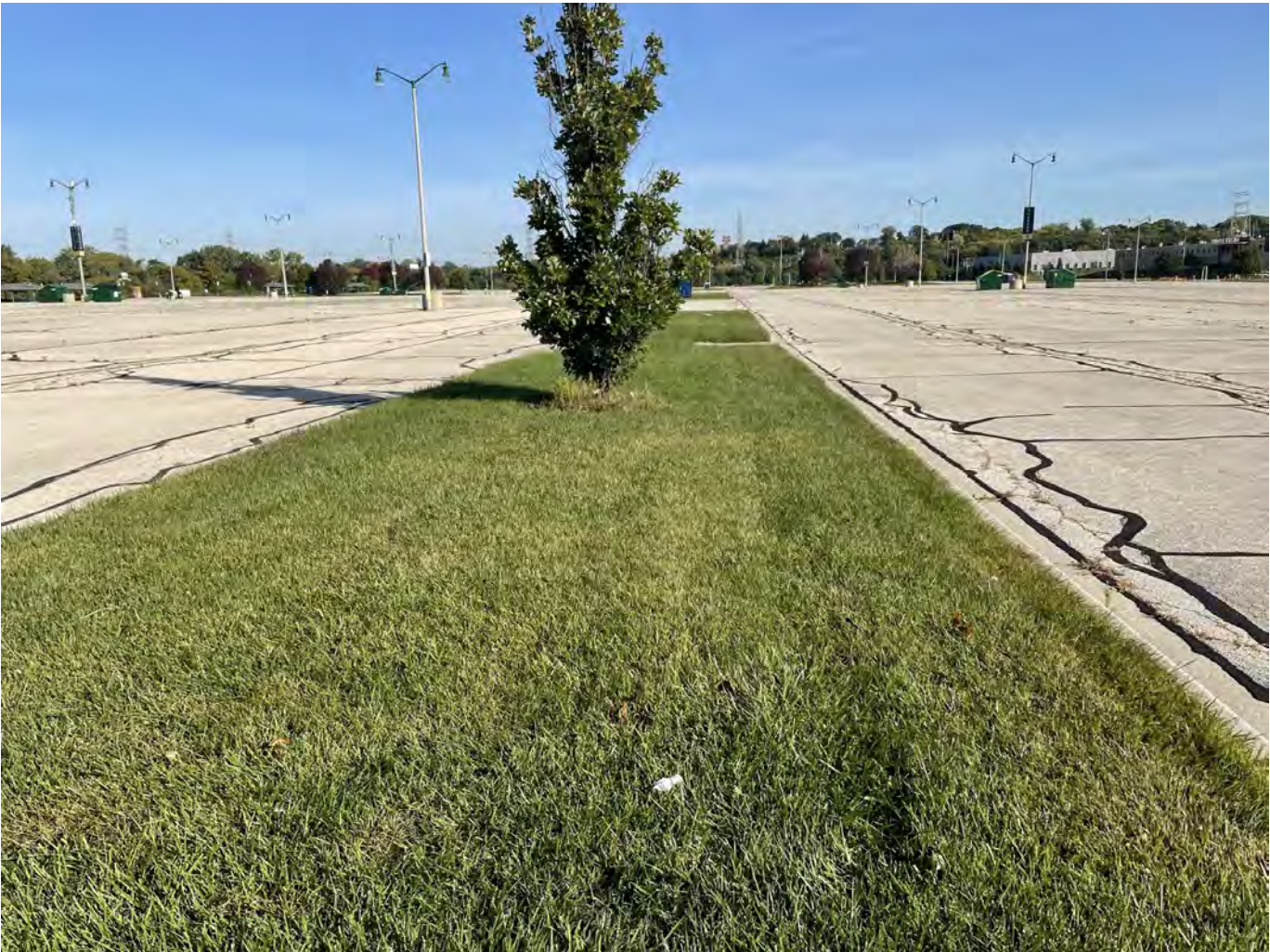
Photo 11: Uecker Lot: Greenspace cap over Uecker Lot island: 12-inches low permeability soil covered with 4-inches of vegetated topsoil. Photo taken facing north on October 4, 2022.
