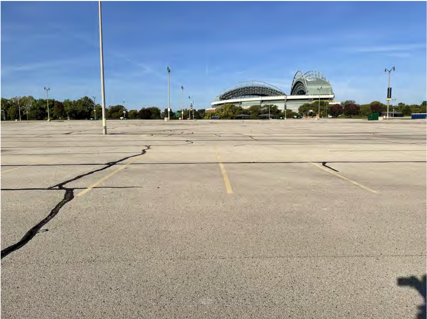
Photo 2: Yount Lot: Asphalt cap over Yount Lot: 4-inch asphalt pavement overlying 8-inches of crushed aggregate base course. Photo depicts current conditions for comparison during future inspections. Photo taken facing west on October 4, 2022.
