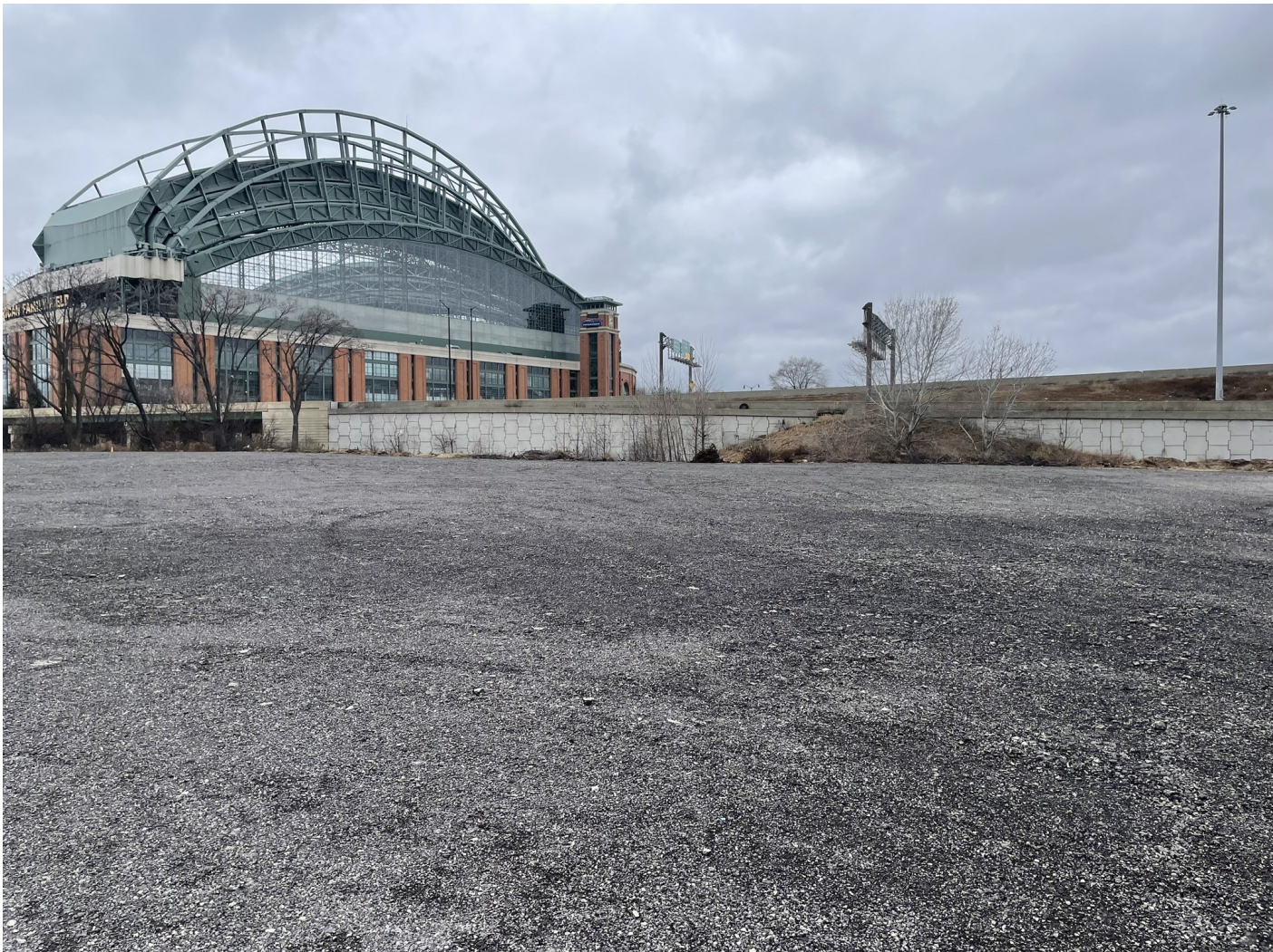
Photo 6: Staff Lot: Compacted milled asphalt cap across the Staff Lot. Between 6 and 12 inches thick. Photo taken facing southwest on January 18, 2023.
