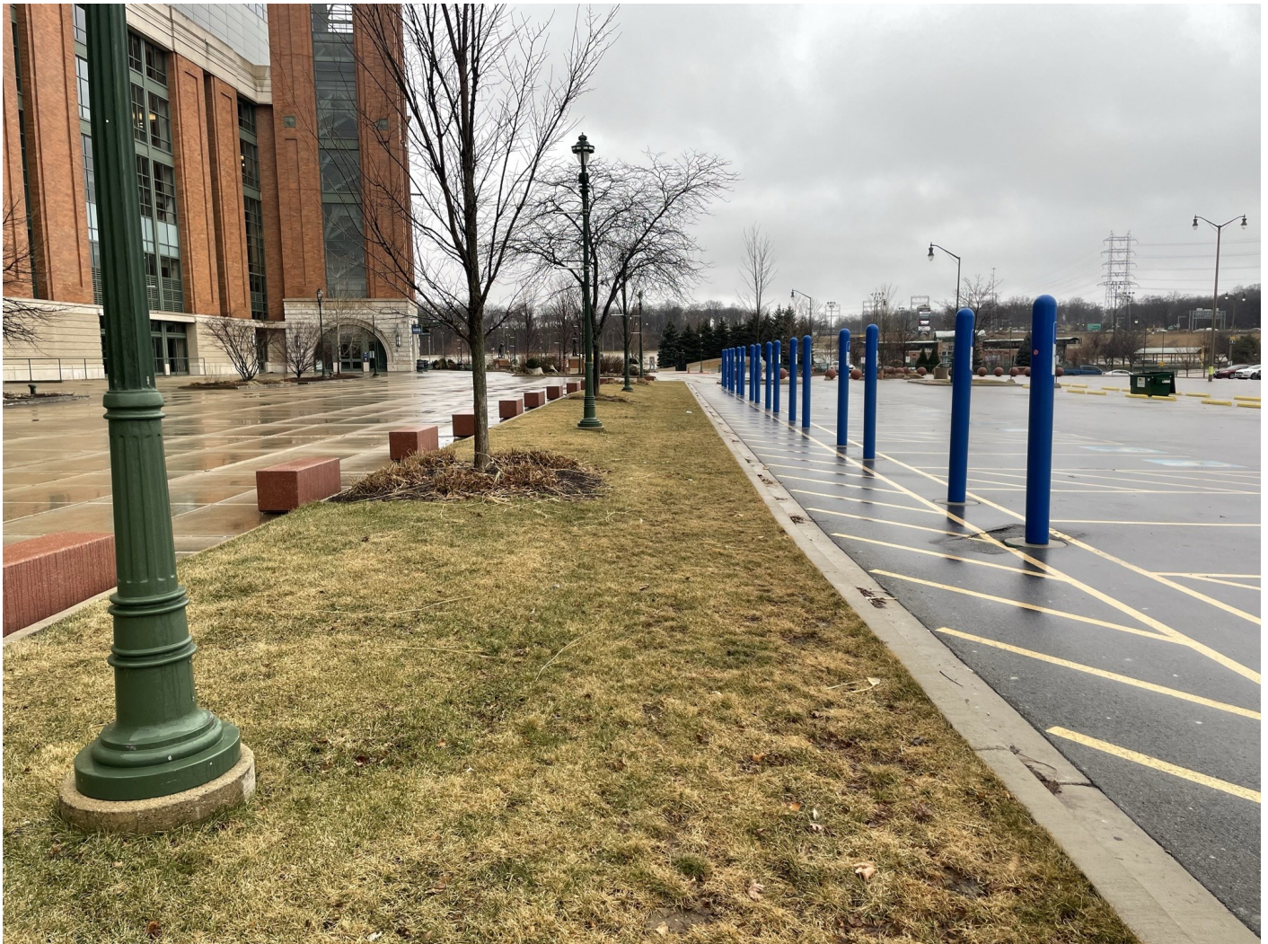
Photo 42: Stadium Plaza area (north side of stadium): Landscaped strip along plaza perimeter. Grass landscaping over 12-inches low permeability non-impacted soil, consistent with islands and medians across the site. Photo taken facing west on January 18, 2023.
