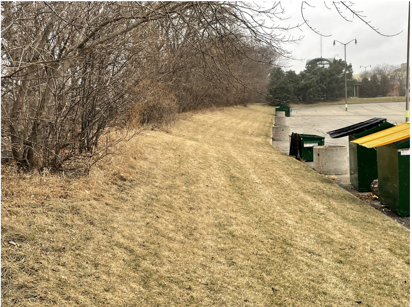
Photo 17: American Family Lot: Greenspace cap along eastern edge of parking lot. 12-inches low permeability non-impacted soil covered with vegetated topsoil. Trees, shrubs, and native plant overgrown shown on left side of photo, which line the Menomonee River banks.
