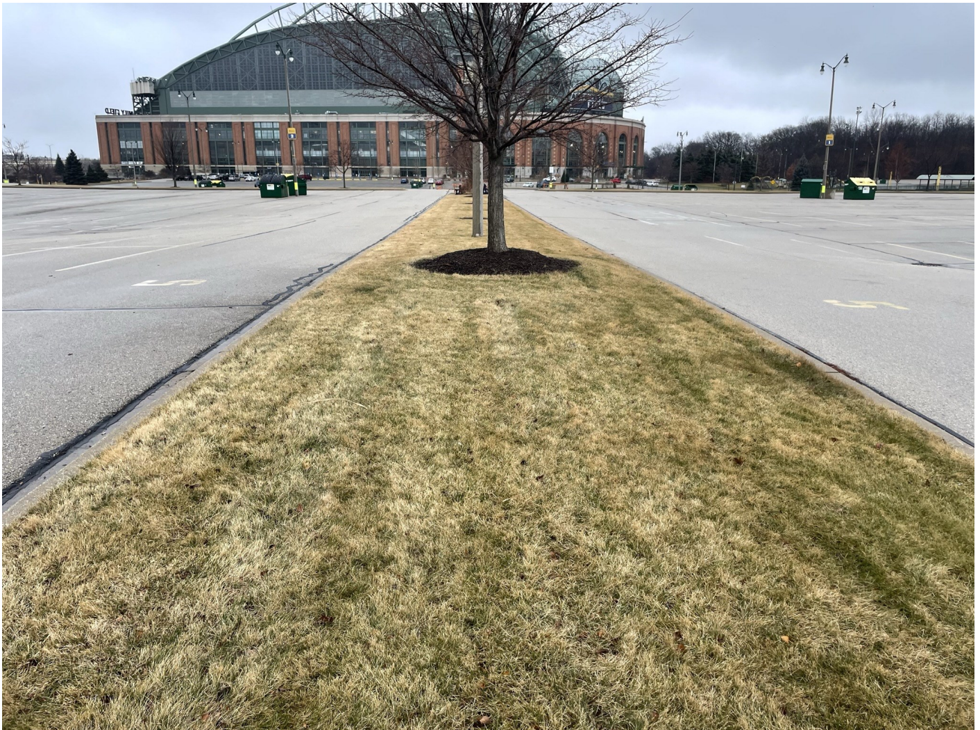
Photo 51: Brewers and Braves Lots plus Selig Drive: Braves 1 (right) and Braves 2 (left) Lots paved with asphalt surface cap: 4-inch asphalt pavement over 8-inches of crushed aggregate. Landscaped greenspace median in central portion of photo: grass topsoil over 12-inches of low permeability non-impacted soil. Photo taken facing south on January 18, 2023.
