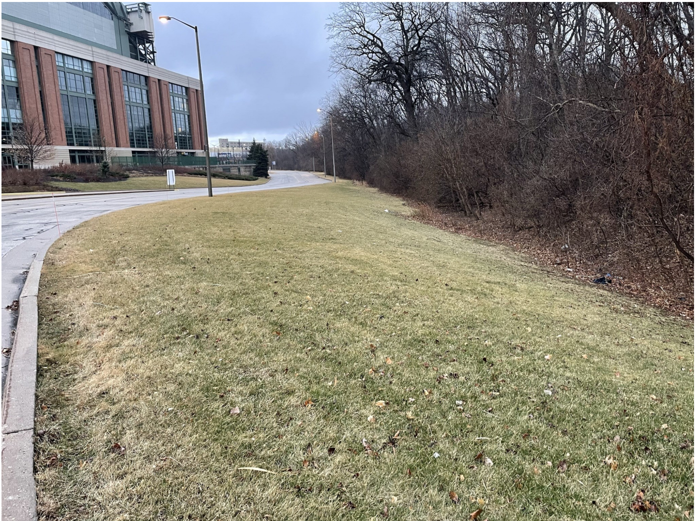
Photo 75: Thomas Lot - Frederick Miller Way: Greenspace cap along the south side of asphalt capped Frederick Miller Way (left). Concrete cap curb and gutter running along the roadway. Photo taken facing southeast on January 18, 2023.
