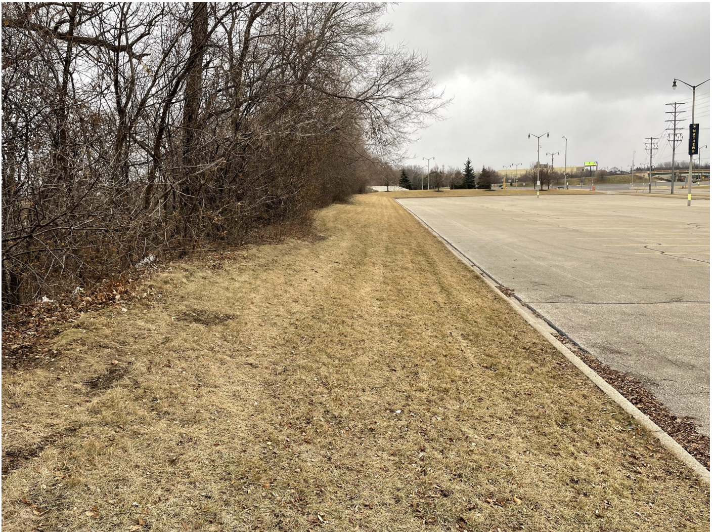
Photo 10: Matthews Lot: Greenspace cap along eastern edge of Matthews Lot, representative of greenspace across the River West site. 12-inch low-permeability non-impacted soil cap covered with vegetated topsoil. Trees and overgrowth shown on left side of photo, which represents the surface cover conditions along the Menomonee River banks on-site. Photo taken facing south on January 18, 2023.
