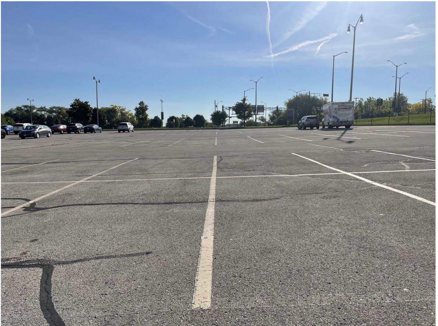
Photo 28: Kuenn Lot: Asphalt cap across Kuenn Lot parking lot, representative of asphalt parking lot caps across the River West site. 4-inch asphalt pavement over 8-inches of crushed aggregate. Photo taken facing east on October 4, 2022.
