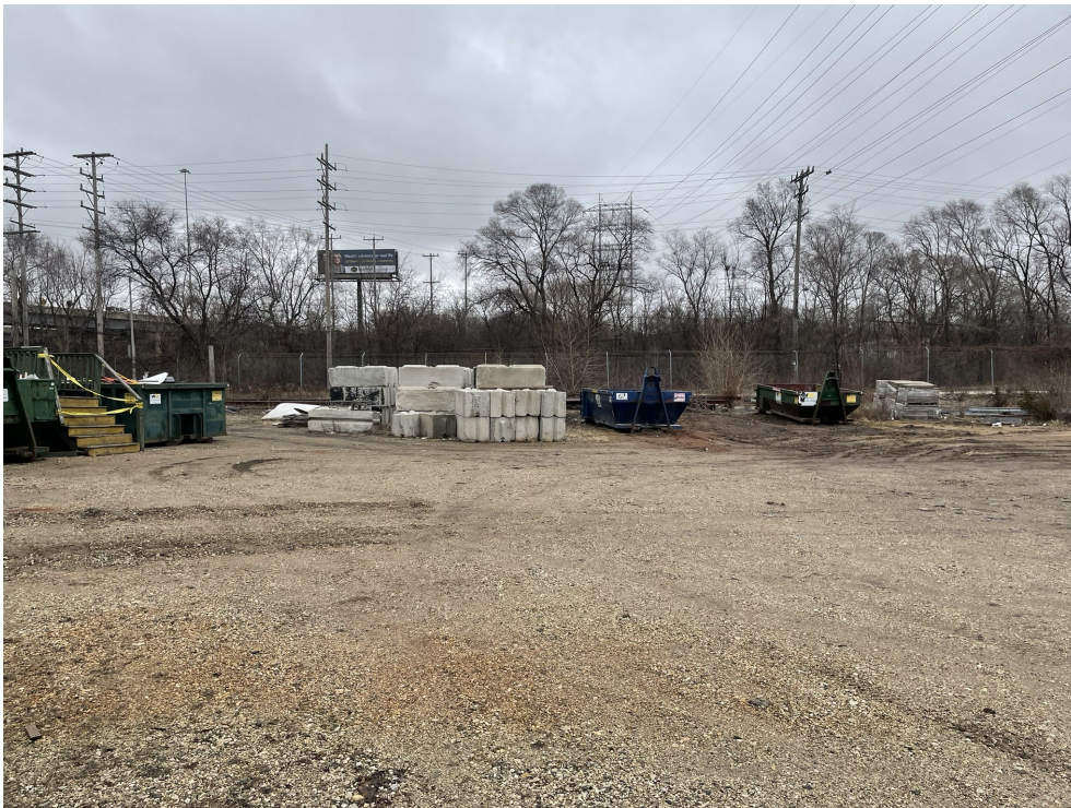
Photo 2: Storage Yard lot: Gravel cap along entrance road consisting of approximately 6-inches of gravel cap over broken asphalt pavement and subgrade. Photo taken facing east on January 18, 2023.
