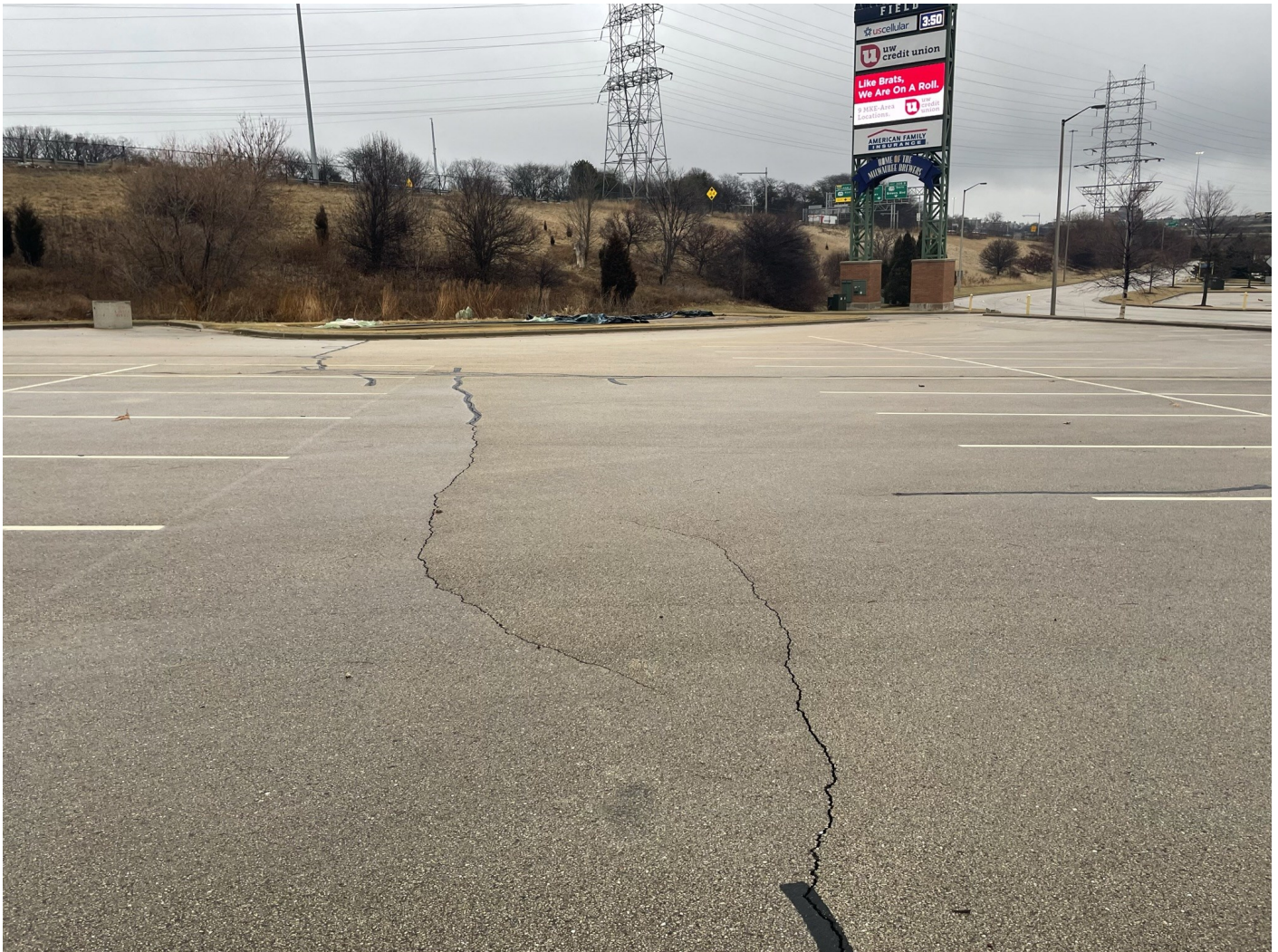
Photo 65: Money Lot - Auxiliary Lot: Asphalt cap surface lot: 4-inch asphalt pavement over 8-inches of crushed aggregate. Photo taken facing east on January 18, 2023.
