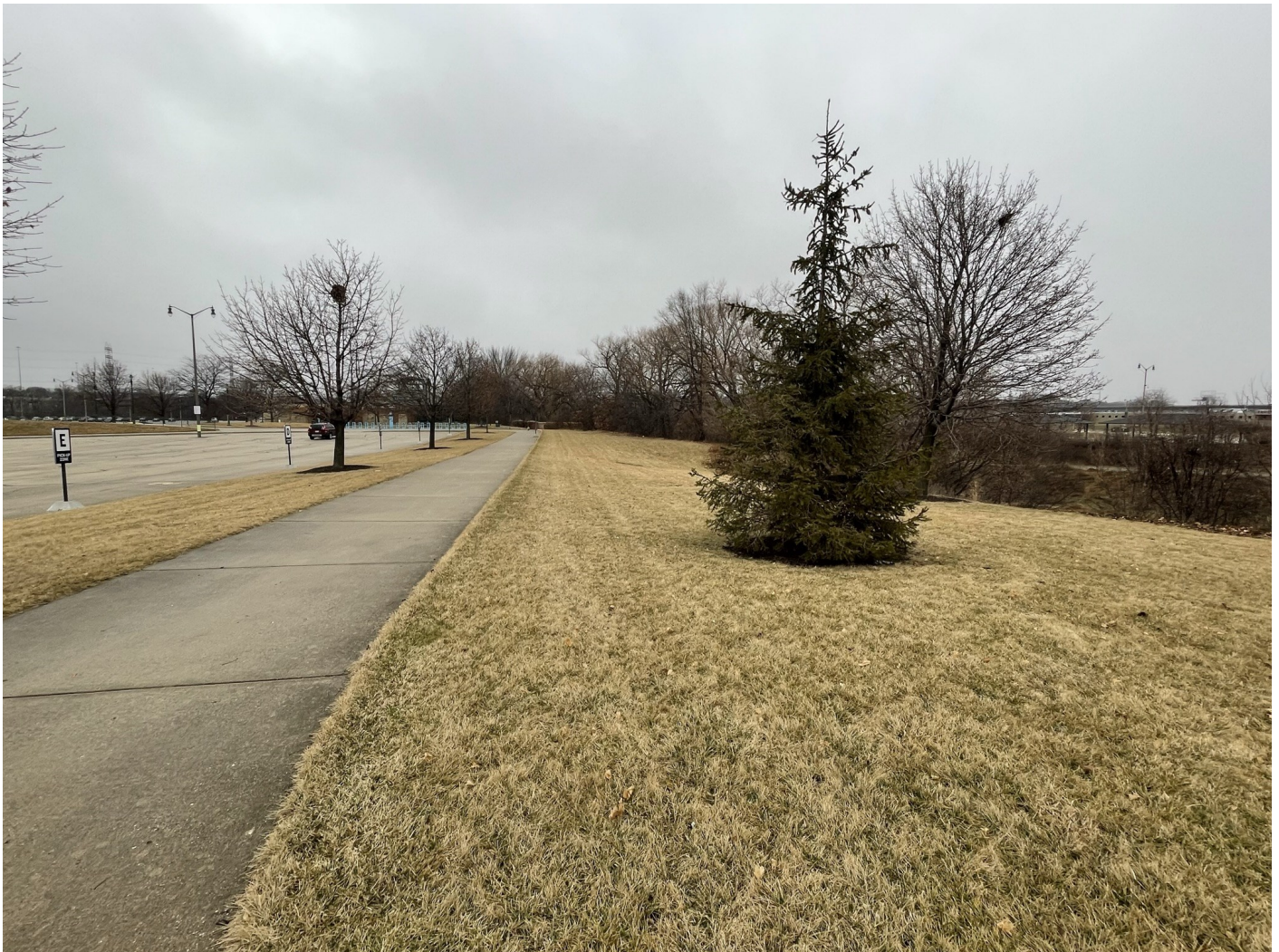
Photo 24: Ganter Lot: Greenspace cap along eastern edge of Ganter Lot. 12-inches low permeability non-impacted soil covered with 4 inches of vegetated topsoil (grass shown here) with various plantings. Asphalt cap pedestrian path shown on left side of photo.
