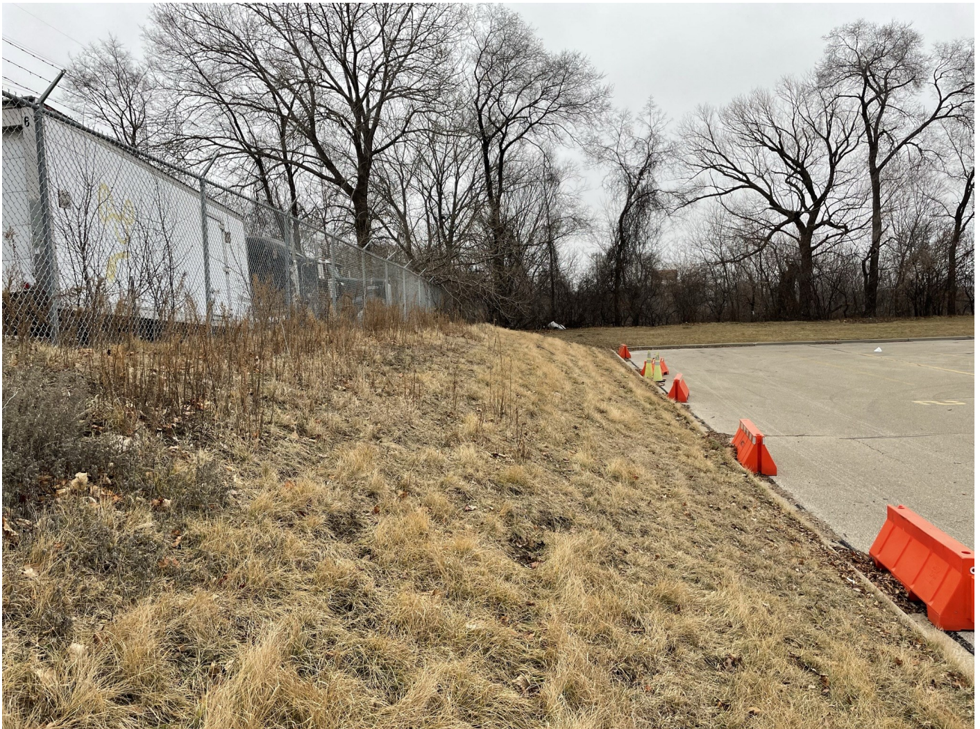
Photo 9: Matthews Lot: Greenspace cap along northern edge of Matthews Lot. 12-inch low-permeability non-impacted soil cap covered with vegetated topsoil. Photo taken facing east on January 18, 2023.
