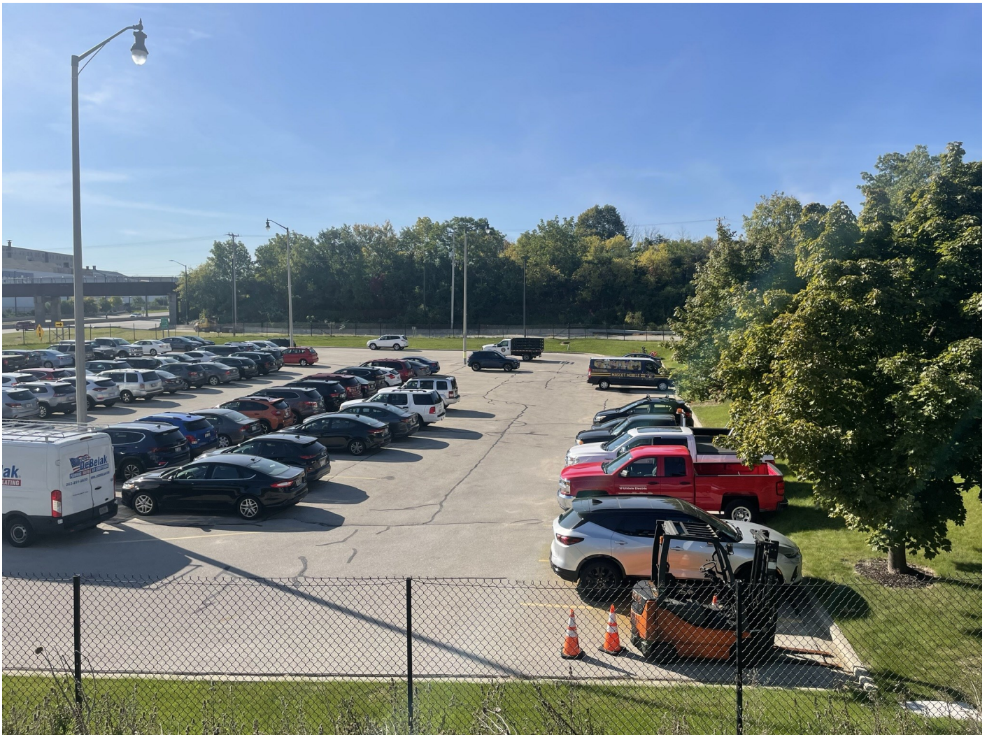
Photo 31: Logan Lot: Asphalt cap across Logan Lot parking lot, representative of asphalt parking lot caps across the River West site. 4-inch asphalt pavement over 8-inches of crushed aggregate. Concrete curb (6-inch thick concrete) and gutter (8-inch thick concrete) over crushed aggregate shown in photo foreground. Greenspace cap shown in photo foreground and on right side of photo: 12-inches of low-permeability non-impacted soil covered with vegetated (grass) topsoil. Photo taken facing south on October 4, 2022.
