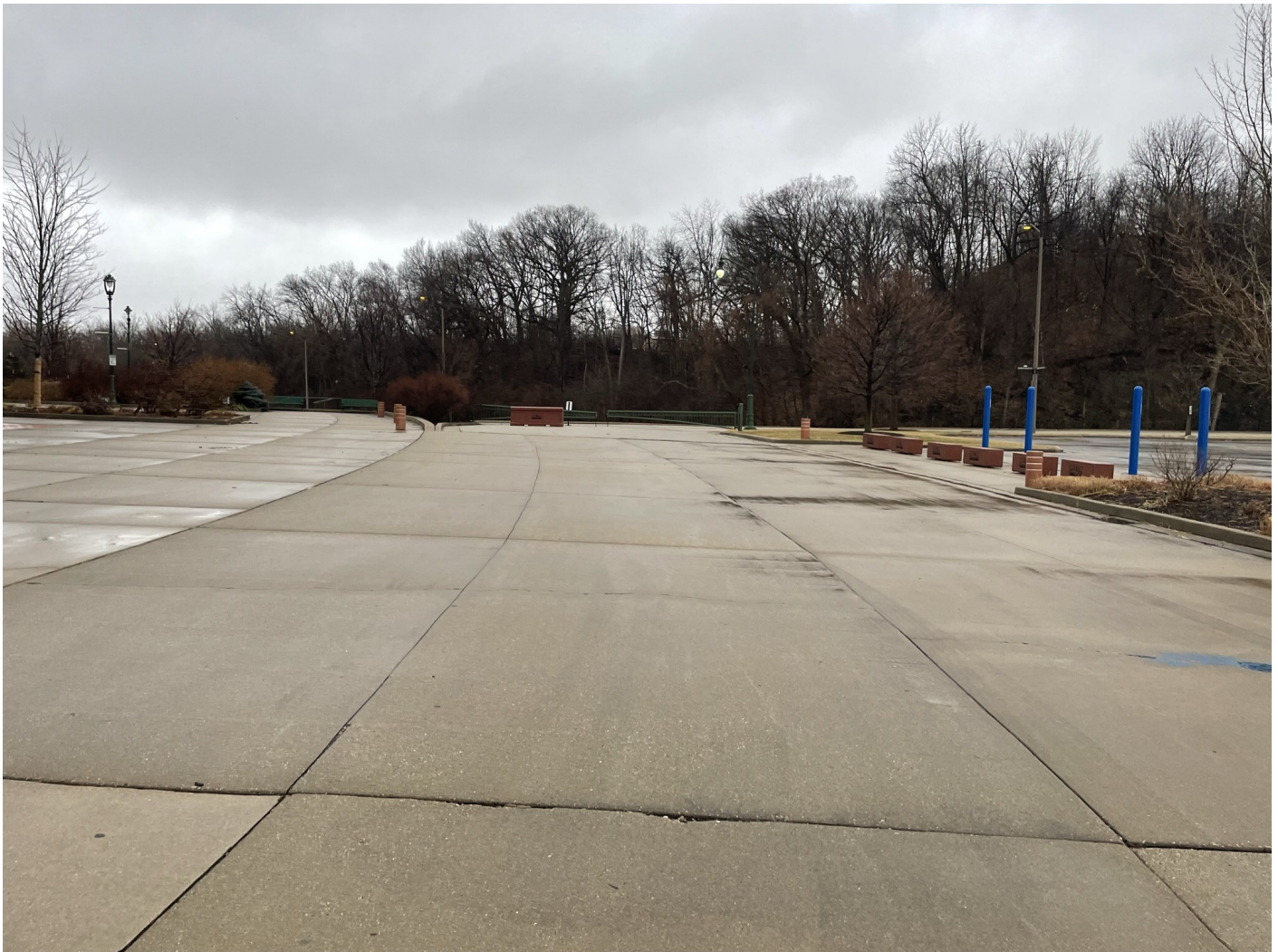
Photo 43: Stadium Plaza area (northwest side of stadium): Concrete pavement cap along exterior plaza sections, Brewers Way, and pedestrian sidewalk. 6-inches of concrete pavement over crushed aggregate. Photo taken facing southwest on January 18, 2023.
