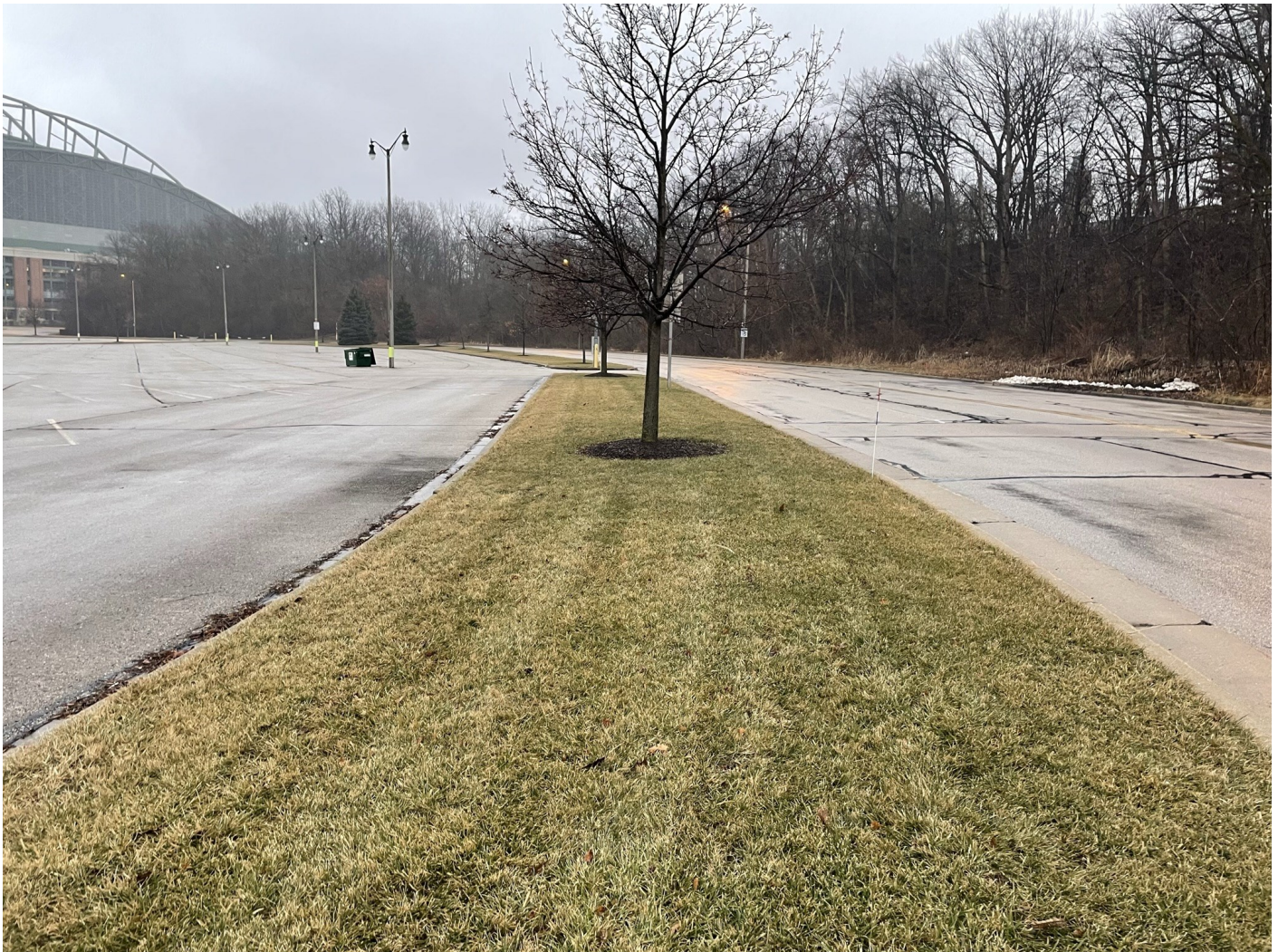
Photo 71: Fingers Lot: Greenspace cap median (center) along the northwest side of asphalt capped Fingers Lot (left), along the east side of asphalt capped Frederick Miller Way (right). Concrete cap curb and gutter running along the median perimeter. Photo taken facing southwest on January 18, 2023.
