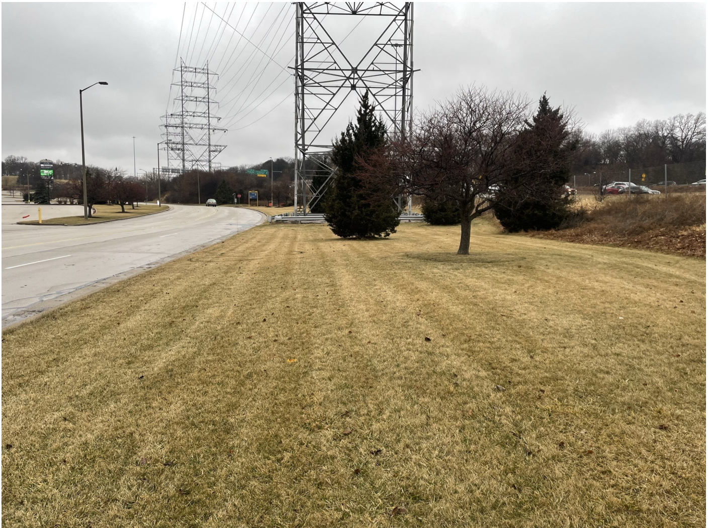
Photo 54: Brewers and Braves Lots plus Selig Drive: Greenspace landscaping along the north side of Selig Drive along Braves Lots. Grass topsoil over 12-inches low permeability non-impacted soil. No ruts or holes in cap. Concrete curb and gutter cap, and asphalt pavement cap along roadway shown in left portion of photo. Photo taken facing west on January 18, 2023.
