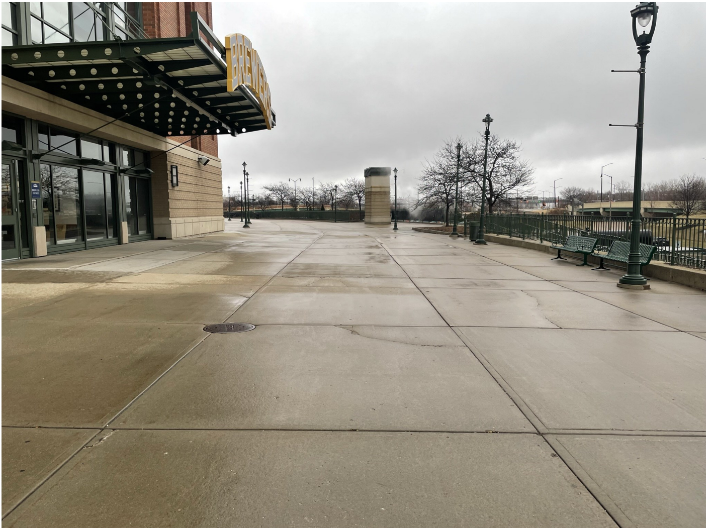
Photo 37: Stadium Plaza area (south side of stadium): Concrete pavement cap along exterior plaza sections and pedestrian sidewalk. 6-inches of concrete pavement over crushed aggregate. Photo taken facing east on January 18, 2023.
