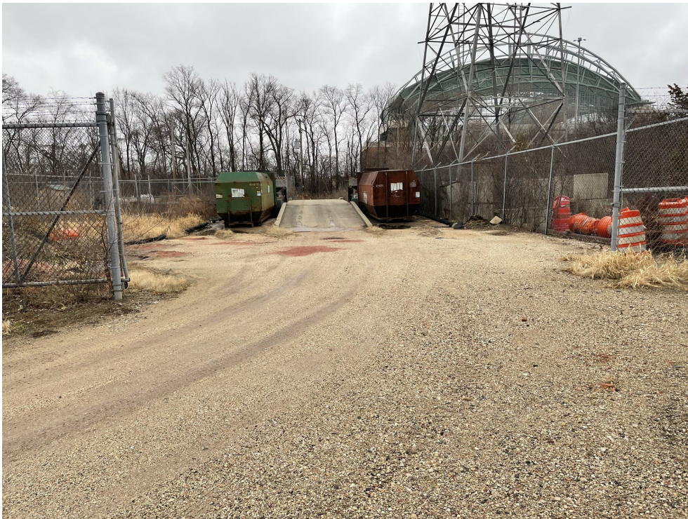
Photo 4: Storage Yard lot: Gravel cap consisting of approximately 6-inches of gravel over broken asphalt pavement and subgrade. Concrete drive pad for disposal vehicles shown in center of photo. Photo taken facing south on January 18, 2023.
