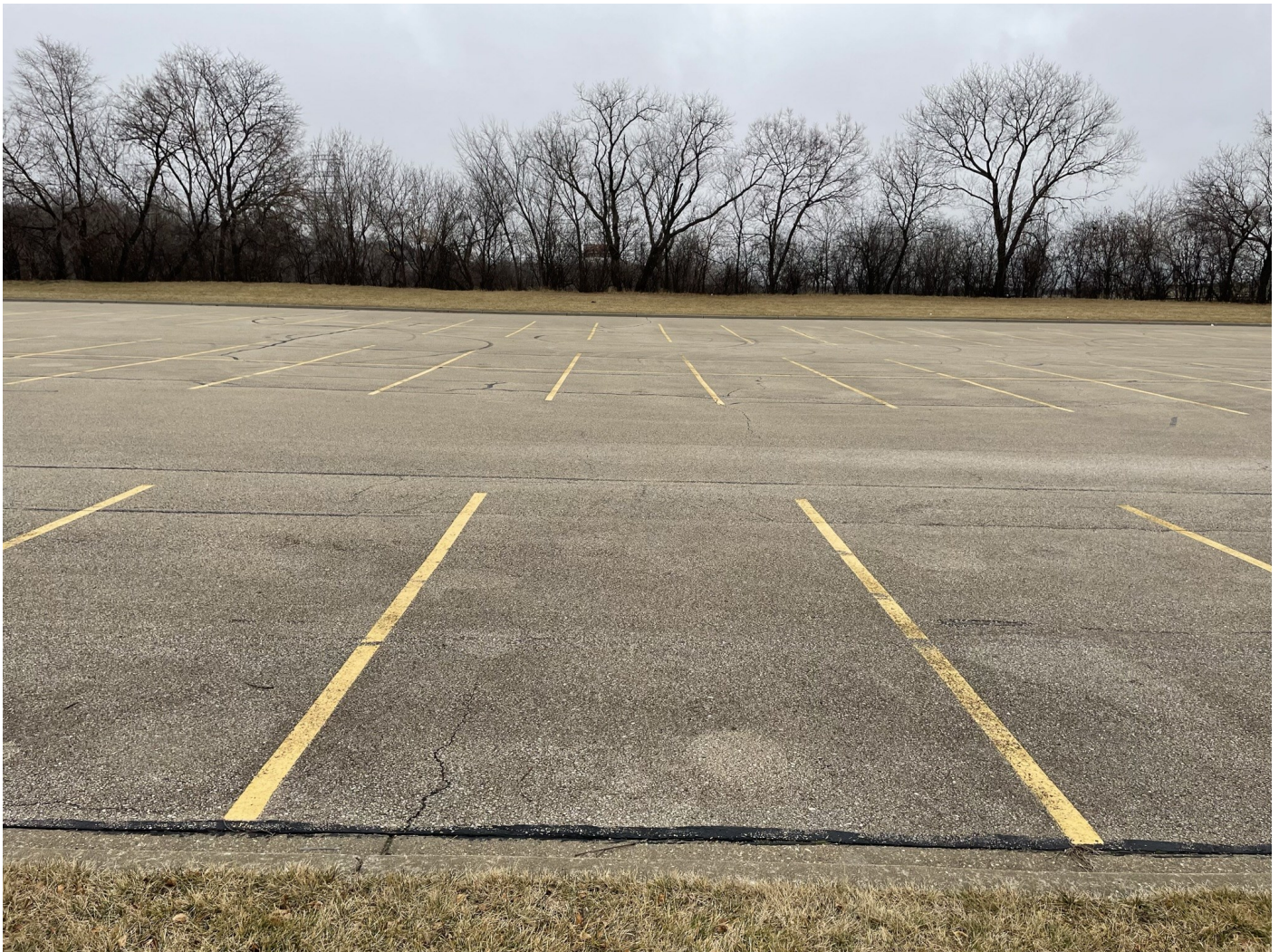
Photo 11: Matthews Lot: Asphalt cap across the entire Matthews Lot parking space, representative of asphalt parking lot caps across the River West site. 4-inch asphalt pavement over 8-inches of crushed aggregate (base course). Photo taken facing east on January 18, 2023.
