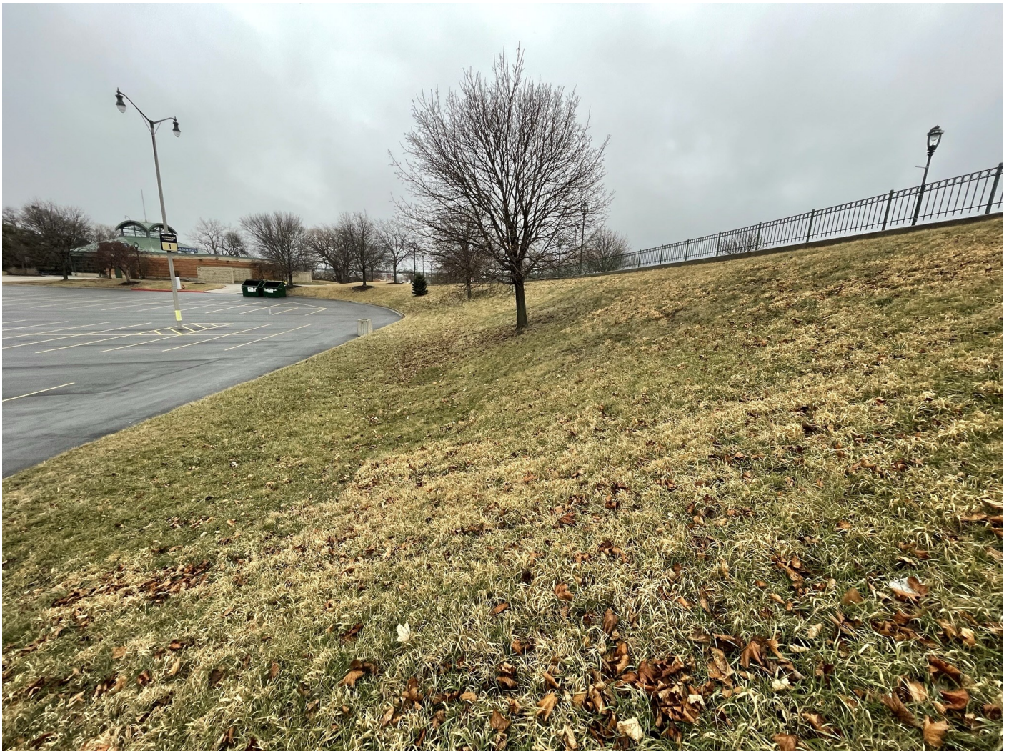
Photo 21: American Family Lot: Greenspace cap along southern edge of parking lot. 12-inches low permeability non-impacted soil covered with vegetated topsoil (grass cover as shown). Photo taken facing east on January 18, 2023.
