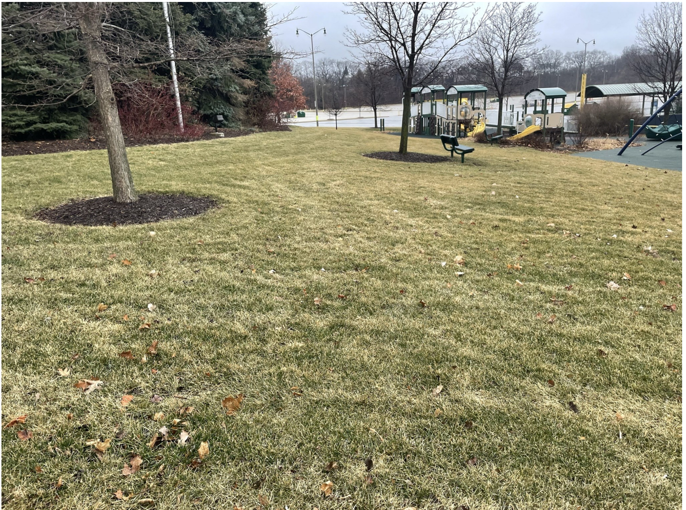
Photo 55: Helfaer Field surrounding areas: Greenspace cap and landscaping cap across playground and grassy hill area southeast of Helfaer Field: Grass or mulch covered topsoil over 12-inches of low permeability non-impacted soil. Photo taken facing west on January 18, 2023.
