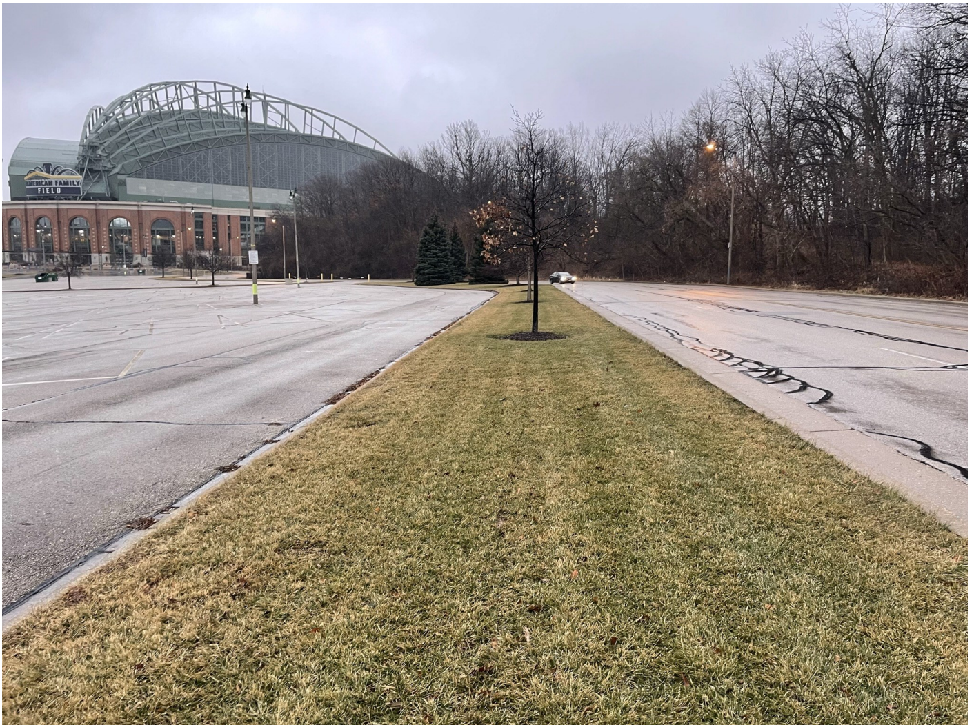
Photo 72: Fingers Lot: Greenspace cap median (center) along the northwest side of asphalt capped Fingers Lot (left), along the east side of asphalt capped Frederick Miller Way (right). Concrete cap curb and gutter running along the median perimeter. Photo taken facing southwest on January 18, 2023.
