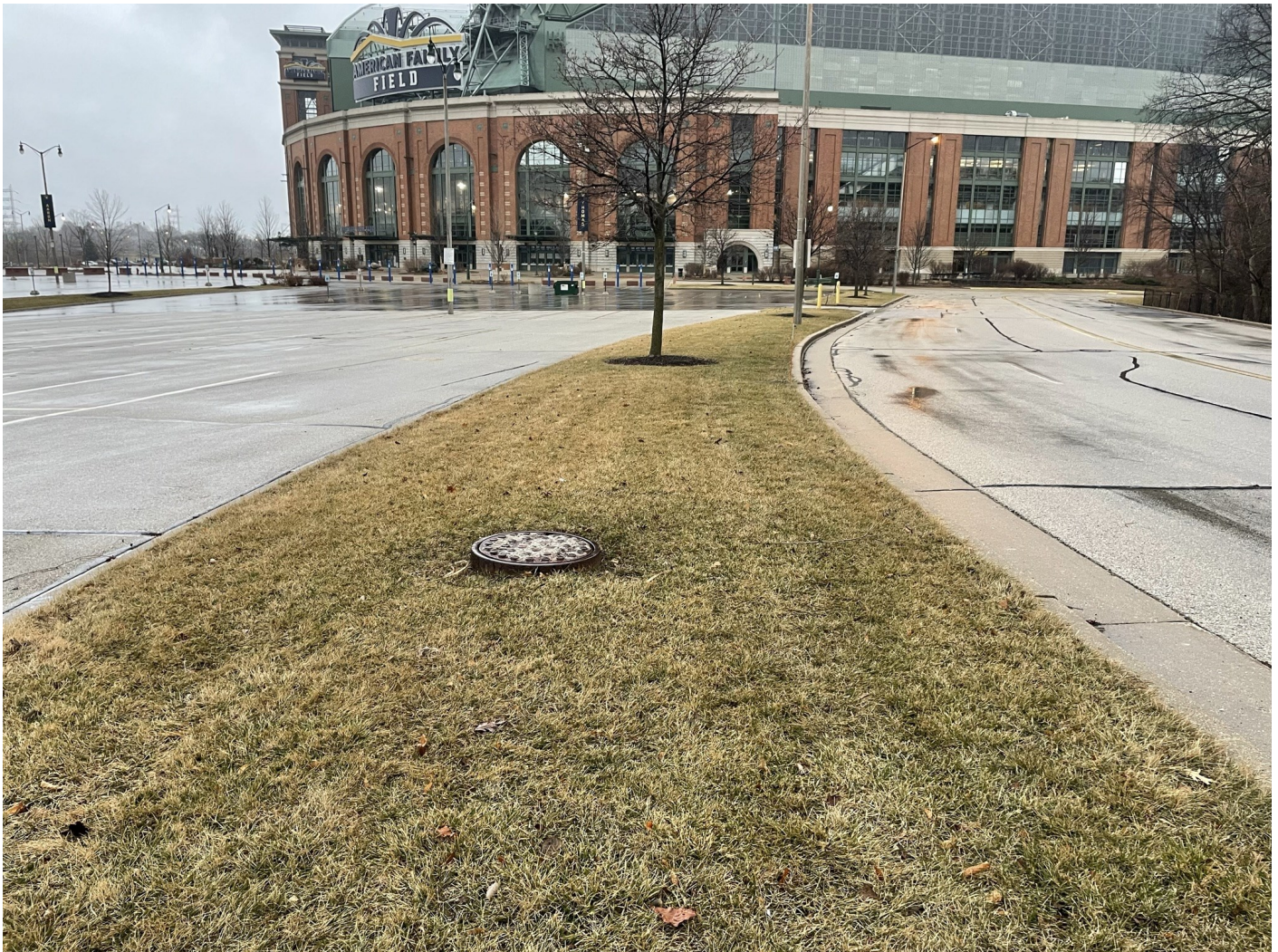
Photo 74: Thomas Lot: Greenspace cap median (center) along the west side of asphalt capped Thomas Lot (left), along the north side of asphalt capped Frederick Miller Way (right). Concrete cap curb and gutter running along the median perimeter. Photo taken facing east on January 18, 2023.
