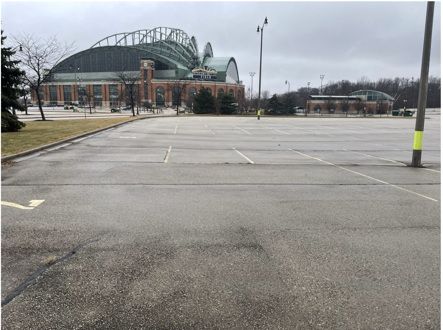
Photo 60: Cooper Lot area: Asphalt cap parking lot: 4-inch asphalt pavement cap over 8-inches of crushed aggregate base course. Photo taken facing south on January 18, 2023.
