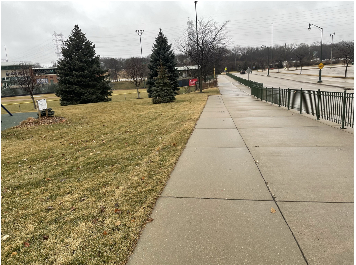
Photo 56: Helfaer Field surrounding areas: Greenspace cap and landscaping cap across playground and grassy hill area southeast of Helfaer Field (left): Grass or mulch covered topsoil over 12-inches of low permeability non-impacted soil. Concrete cap sidewalk along entrance road and east side of Helfaer Field (right): 6-inch concrete cap over 8-inches of crushed aggregate. Photo taken facing north on January 18, 2023.
