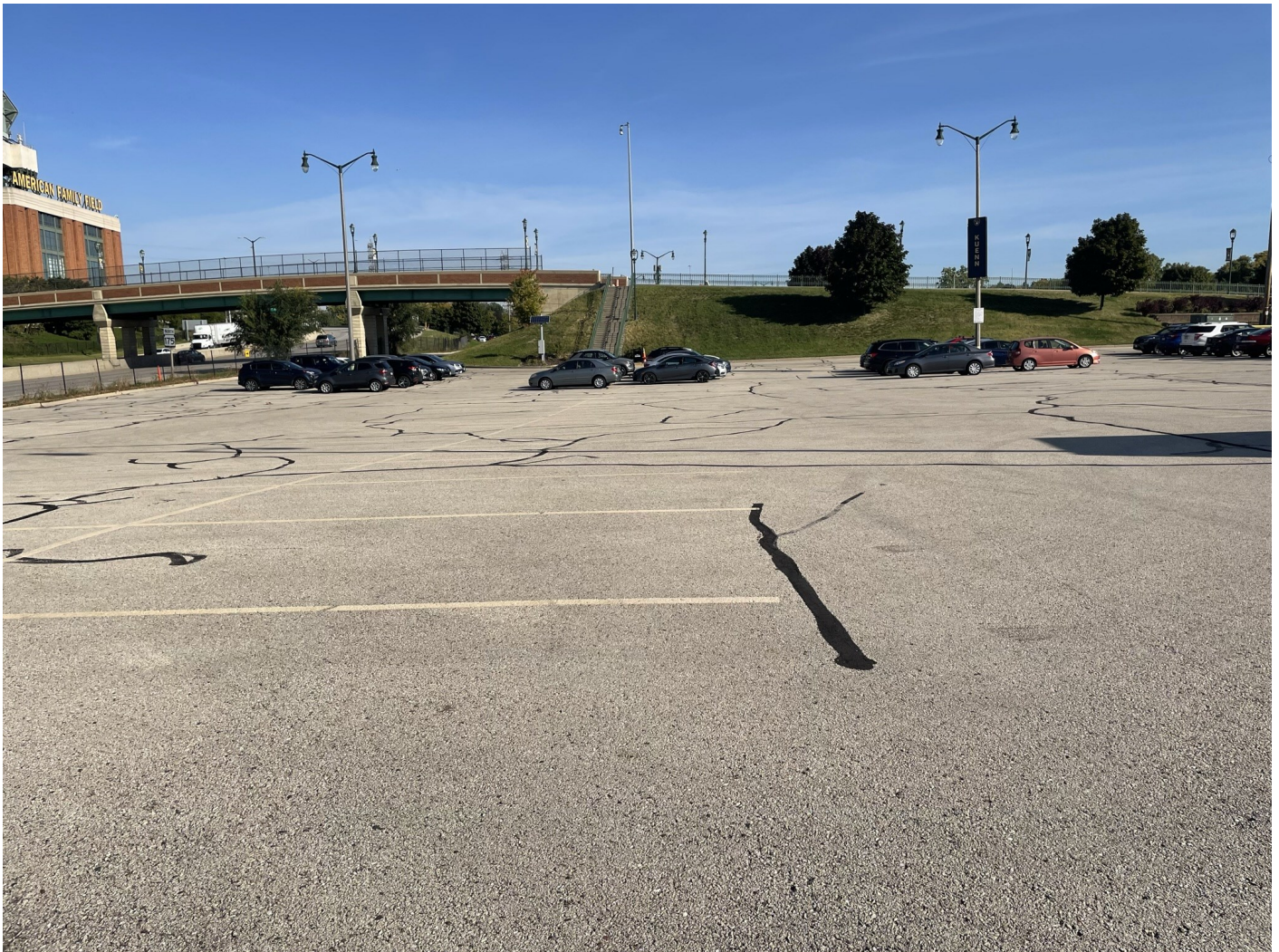
Photo 29: Kuenn Lot: Asphalt cap across Kuenn Lot parking lot, representative of asphalt parking lot caps across the River West site. 4-inch asphalt pavement over 8-inches of crushed aggregate. Photo taken facing north on October 4, 2022.
