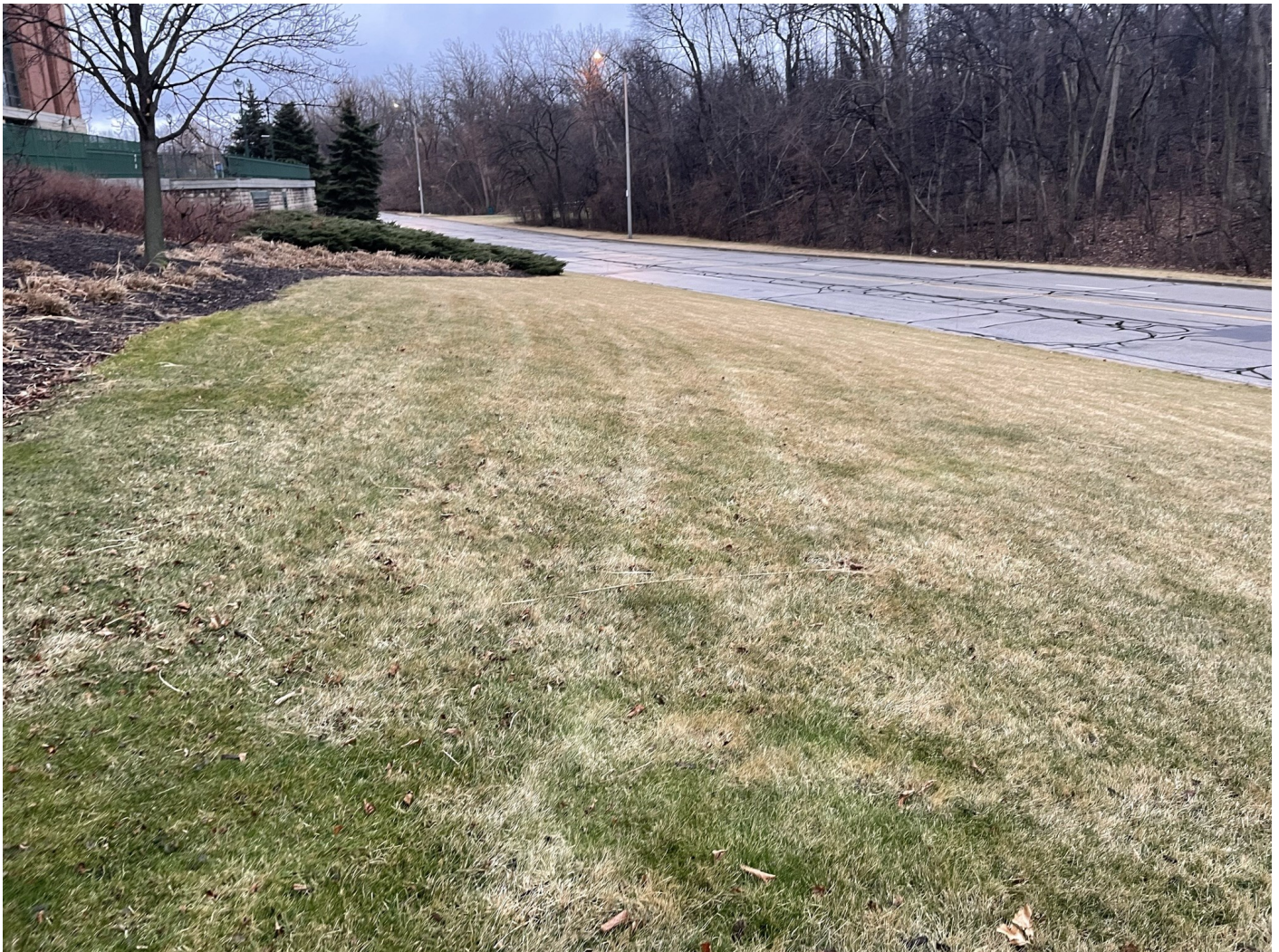
Photo 44: Stadium Plaza area (west side of stadium): Landscaping cap along west side of stadium plaza and east side of Frederick Miller Way: Grass landscaping over 12-inches low permeability non-impacted soil, consistent with greenspace across the site. Frederick Miller Way capped with asphalt pavement cap. Photo taken facing south on January 18, 2023.
