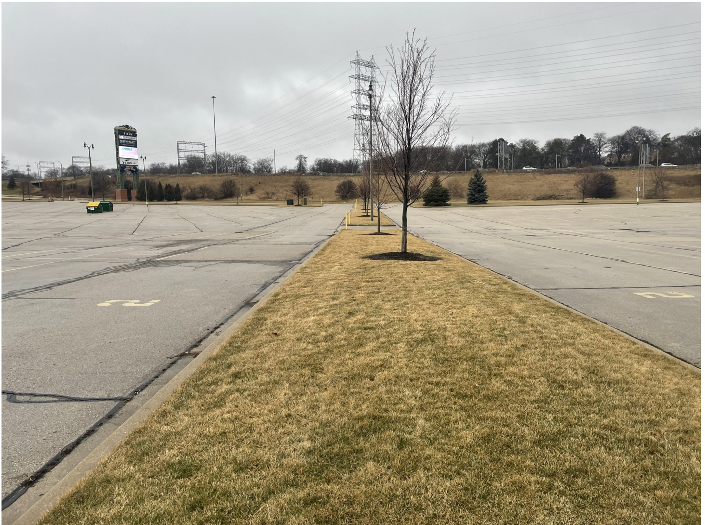
Photo 62: Cooper Lot area: Greenspace cap median between Cooper Lot and Money Lot. Asphalt capped lots on left and right side of greenspace cap median in center of photo. Photo taken facing northwest on January 18, 2023.
