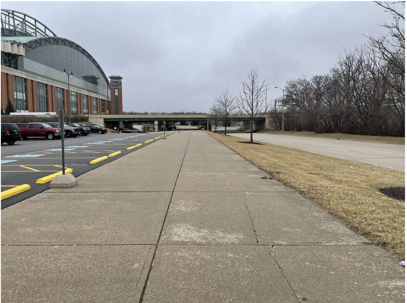
Photo 13: American Family Lot: Concrete pedestrian path cap along northern edge of the lot. 6-inches of concrete pavement over 8-inches of crushed aggregate. Asphalt parking lot cap shown on left side of photo. Greenspace cap shown on right side of photo. Selig Drive on far right side of photo, asphalt pavement cap same construction as asphalt parking lot space. Photo taken facing west on January 18, 2023.
