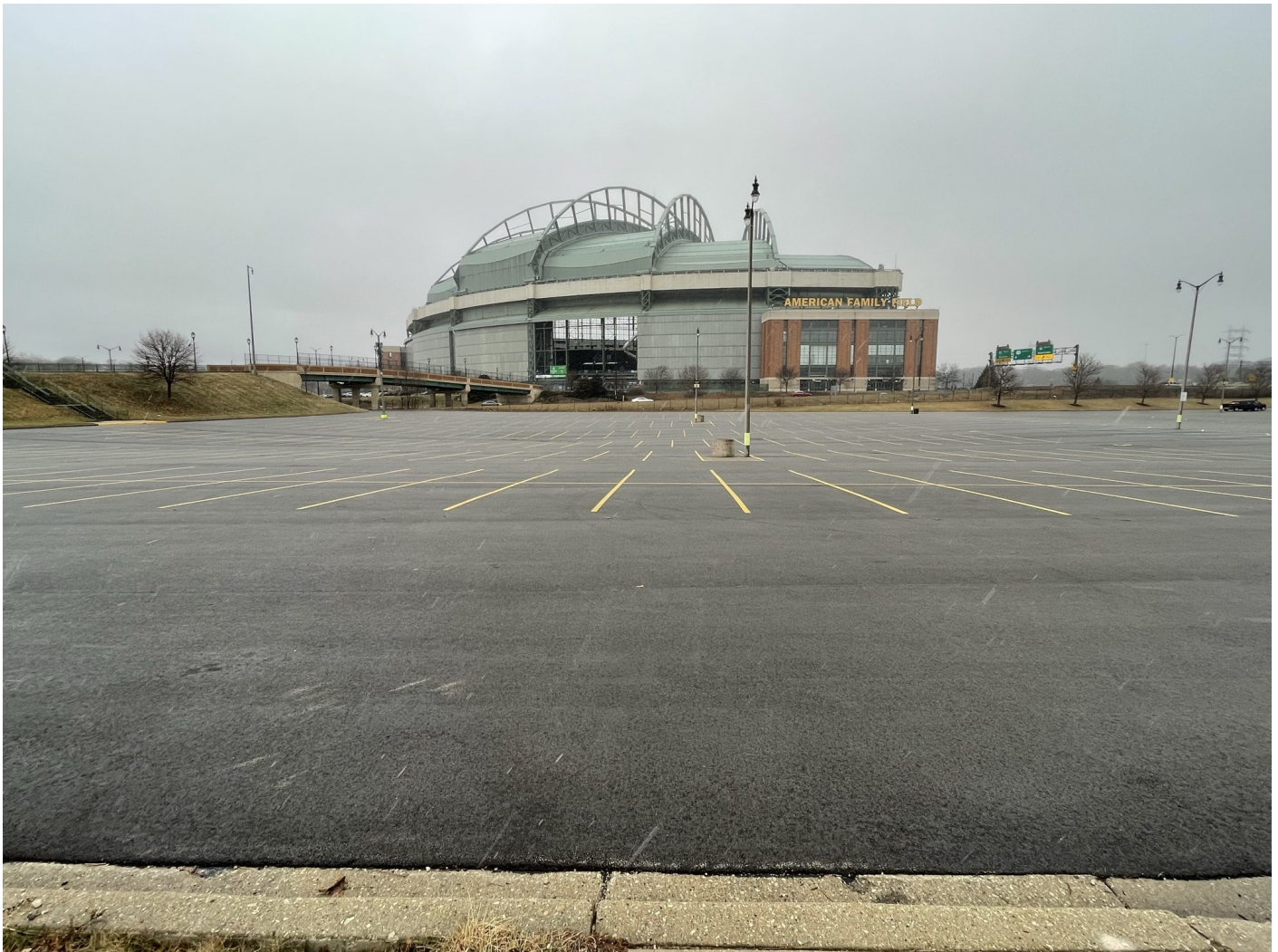
Photo 20: American Family Lot: Asphalt capped surface parking lot (American Family Lot). 4-inches of asphalt pavement over 8-inches of crushed aggregate. Concrete curb and gutter shown in photo foreground, consisting of 6-inch thick concrete (curb) or 8-inch thick concrete (gutter) over crushed aggregate base. Photo taken facing west on January 18, 2023.
