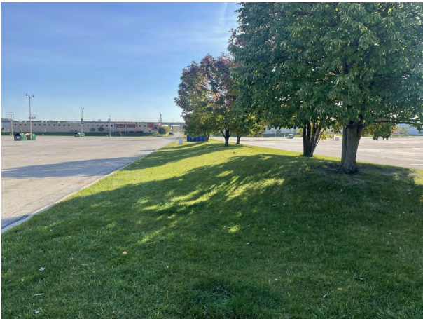
Photo 19: Uecker/Yount Lot: Greenspace cap parking lot island/median between Yount and Uecker Lots on west side of site: 12-inches of low permeability non-impacted soil covered with 4-inches of vegetated topsoil (grass) as well as various landscape plantings. Photo taken facing east on October 4, 2022.
