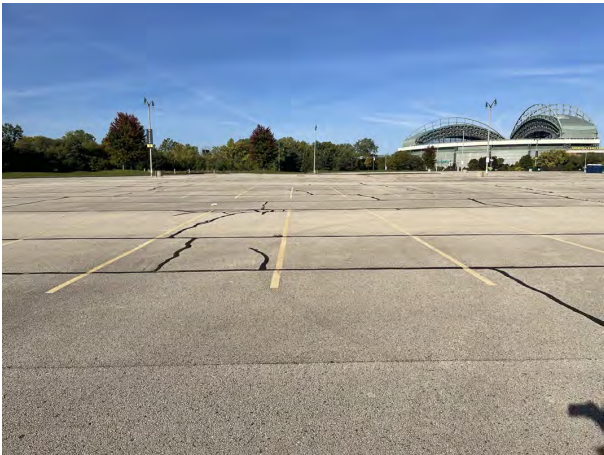
Photo 7: Uecker Lot: Asphalt cap over Uecker Lot: 4-inch asphalt pavement overlying 8-inches of crushed aggregate base course. Photo taken facing west on October 4, 2022.
