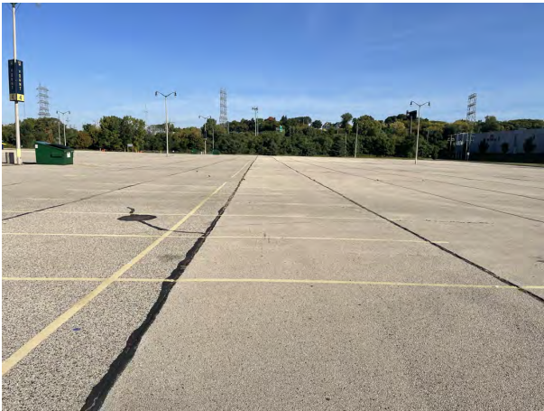
Photo 28: Yount Lot: Asphalt cap over Yount Lot: 4-inch asphalt pavement overlying 8-inches of crushed aggregate base course. Photo taken facing north on October 4, 2022.
