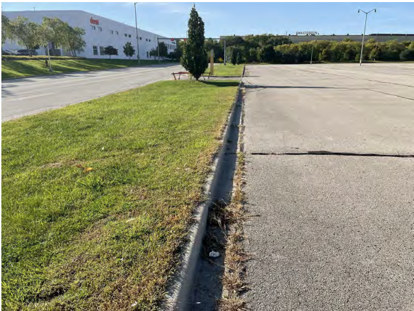
Photo 3: Yount Lot: Asphalt cap over Yount Lot (right side of photo): 4-inch asphalt pavement overlying 8-inches of crushed aggregate base course. Greenspace cap over parking lot median: 12-inches of low-permeability non-impacted soil covered with 4-inches of vegetated topsoil. Concrete curb and gutter along median perimeter and edge of asphalt pavement. Photo taken facing south on October 4, 2022.
