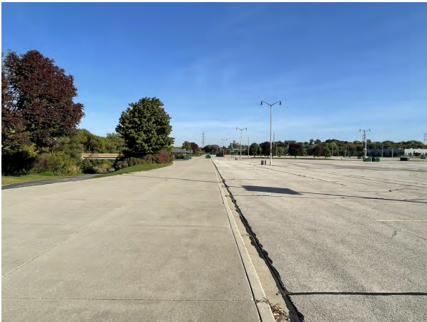
Photo 15: Uecker Lot: Concrete paved plaza and pedestrian path along west side of Uecker Lot (shown on left side of photo): 6-inch concrete pavement overlying 8-inches crushed aggregate. Asphalt paved Uecker Lot (shown on right side of photo): 4-inch asphalt pavement overlying 8-inches crushed aggregate. Photo taken facing north on October 4, 2022.
