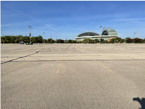
Photo 4: Yount Lot: Asphalt cap over Yount Lot: 4-inch asphalt pavement overlying 8-inches of crushed aggregate base course. Photo depicts current conditions for comparison during future inspections. Photo taken facing west on October 4, 2022.
