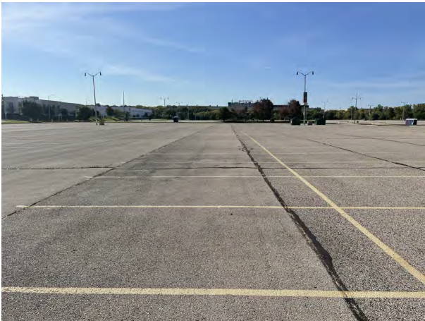
Photo 27: Yount Lot: Asphalt cap over Yount Lot: 4-inch asphalt pavement overlying 8-inches of crushed aggregate base course. Photo taken facing south on October 4, 2022.
