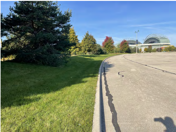
Photo 8: Uecker Lot: Asphalt cap over Uecker Lot (right side of photo): 4-inch asphalt pavement overlying 8-inches of crushed aggregate base course. Greenspace cap over parking lot median along Frederick Miller Way on south side of Uecker Lot: 12-inches of low-permeability non-impacted soil covered with 4-inches of vegetated topsoil. Concrete curb and gutter along median perimeter and edge of asphalt pavement. Photo taken facing west-northwest on October 4, 2022.
