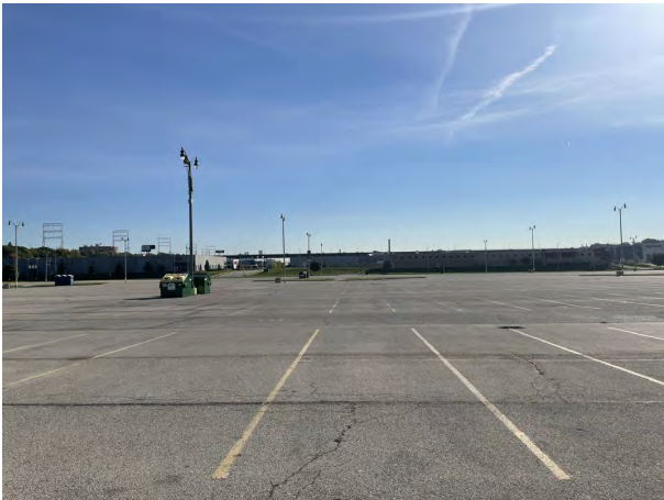
Photo 20: Yount Lot: Asphalt cap over Yount Lot: 4-inch asphalt pavement overlying 8-inches of crushed aggregate base course. Photo taken facing east on October 4, 2022.
