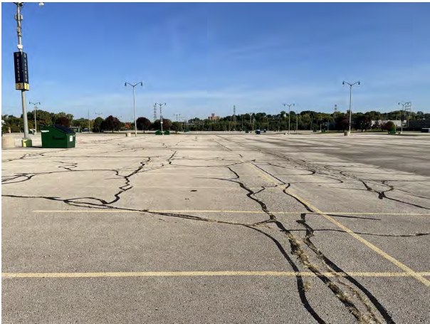
Photo 12: Uecker Lot: Asphalt cap over Uecker Lot: 4-inch asphalt pavement overlying 8-inches of crushed aggregate base course. Photo taken facing north on October 4, 2022.
