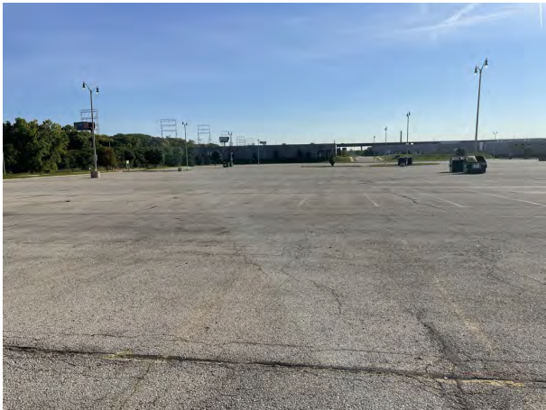
Photo 21: Yount Lot: Asphalt cap over Yount Lot: 4-inch asphalt pavement overlying 8-inches of crushed aggregate base course. Photo taken facing east on October 4, 2022.
