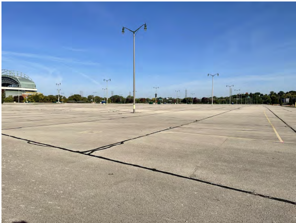
Photo 9: Uecker Lot: Asphalt cap over Uecker Lot: 4-inch asphalt pavement overlying 8-inches of crushed aggregate base course. Photo taken facing northwest on October 4, 2022.
