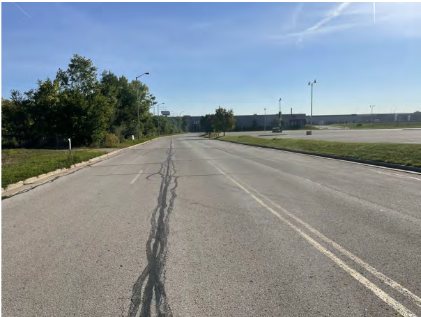
Photo 25: Yount Lot: Asphalt cap over Selig Drive north of Yount Lot: 4-inch asphalt pavement overlying 8-inches of crushed aggregate base course. Photo taken facing east on October 4, 2022.
