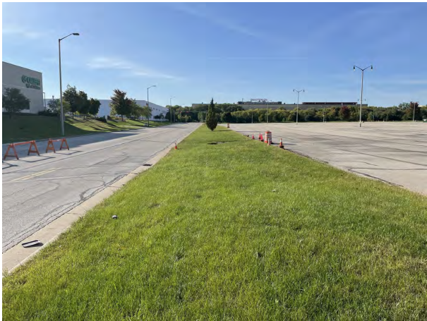
Photo 1: Yount Lot: Greenspace cap along parking lot median: 12-inches of low permeability non-impacted soil covered with 4-inches of vegetated (grass as shown) topsoil. Asphalt capped Selig Drive shown on left side of photo. Asphalt capped Yount Lot shown on right side of photo. Photo taken facing south on October 4, 2022.
