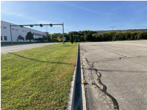
Photo 5: Uecker Lot: Asphalt cap over Uecker Lot (right side of photo): 4-inch asphalt pavement overlying 8-inches of crushed aggregate base course. Greenspace cap over parking lot median: 12-inches of low-permeability non-impacted soil covered with 4-inches of vegetated topsoil. Concrete curb and gutter along median perimeter and edge of asphalt pavement. Photo taken facing south on October 4, 2022.
