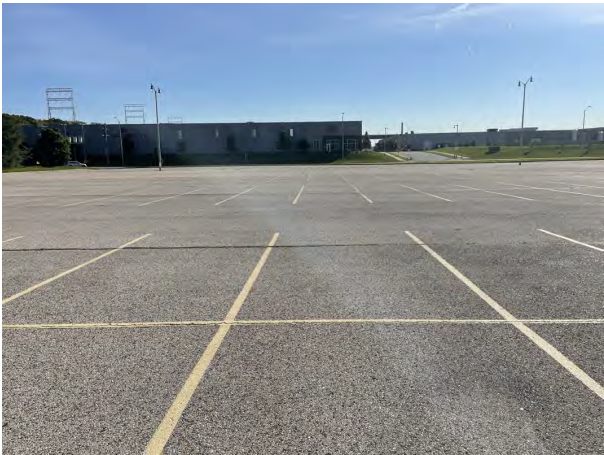
Photo 26: Yount Lot: Asphalt cap over Yount Lot: 4-inch asphalt pavement overlying 8-inches of crushed aggregate base course. Photo taken facing east on October 4, 2022.
